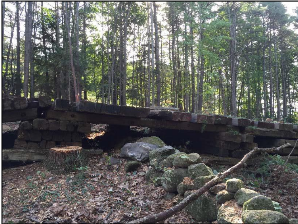
Figure 1. Timber Matting Over Stone Wall Segment
