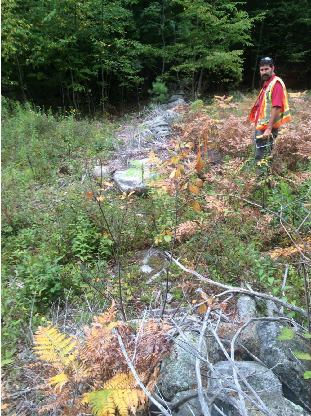
Northern stone wall alignment facing east showing location of breach and carpet of moss on rocks forming the base of the breach.
