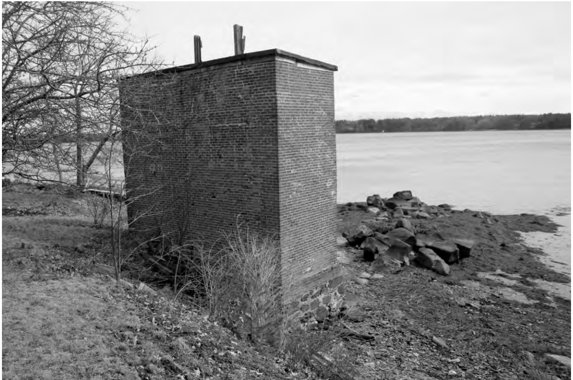
Photo 8) Durham Cable House
