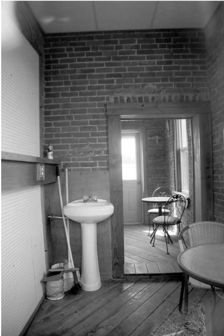
Photo 5) Partition wall (former exterior wall) interior Newington Cable House
