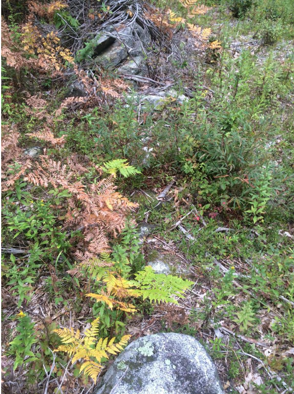
Northern stone wall alignment facing west showing location of breach and growth of a carpet of moss on rocks forming the base of the breach.
