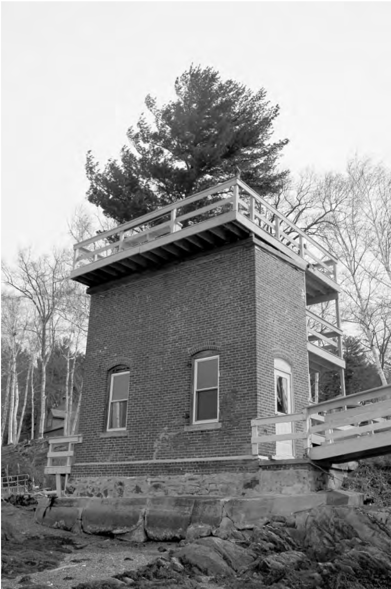
Photo 2) Newington Cable House, from Little Bay shore
