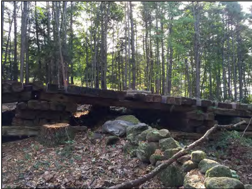
Figure 1. Timber Matting Over Stone Wall Segment
