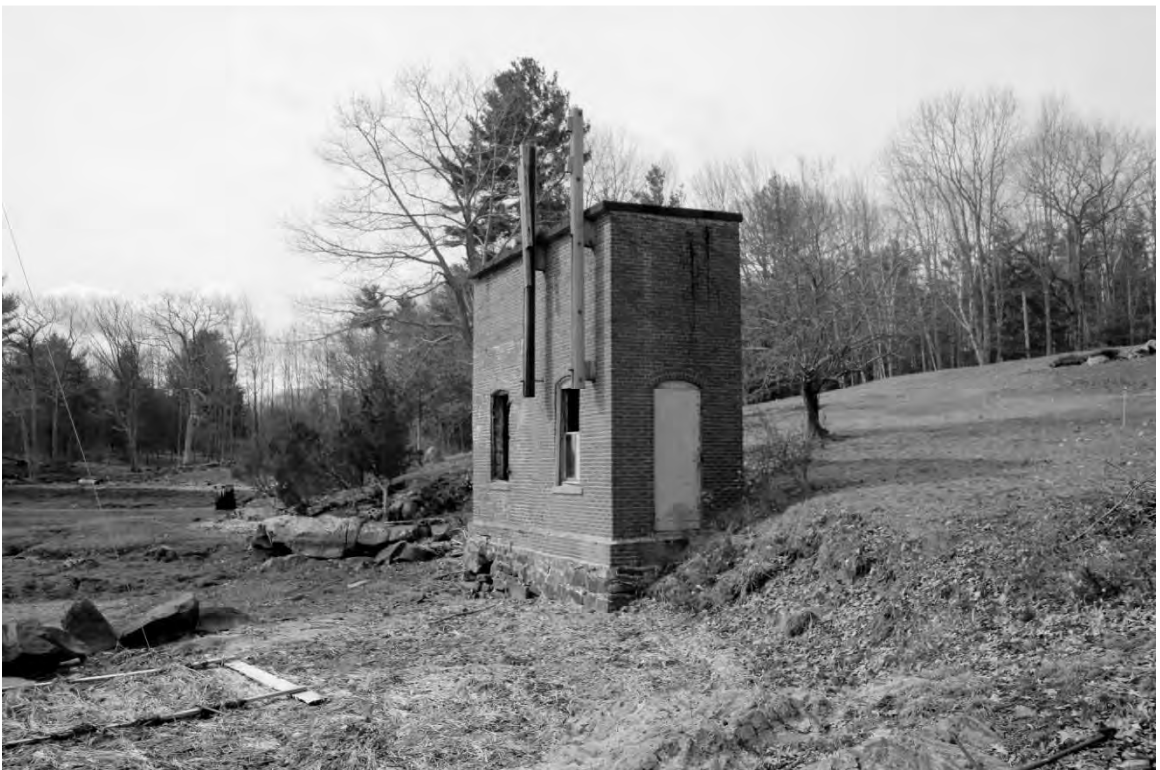
Photo 7) Durham Cable House, from shore of Little Bay
