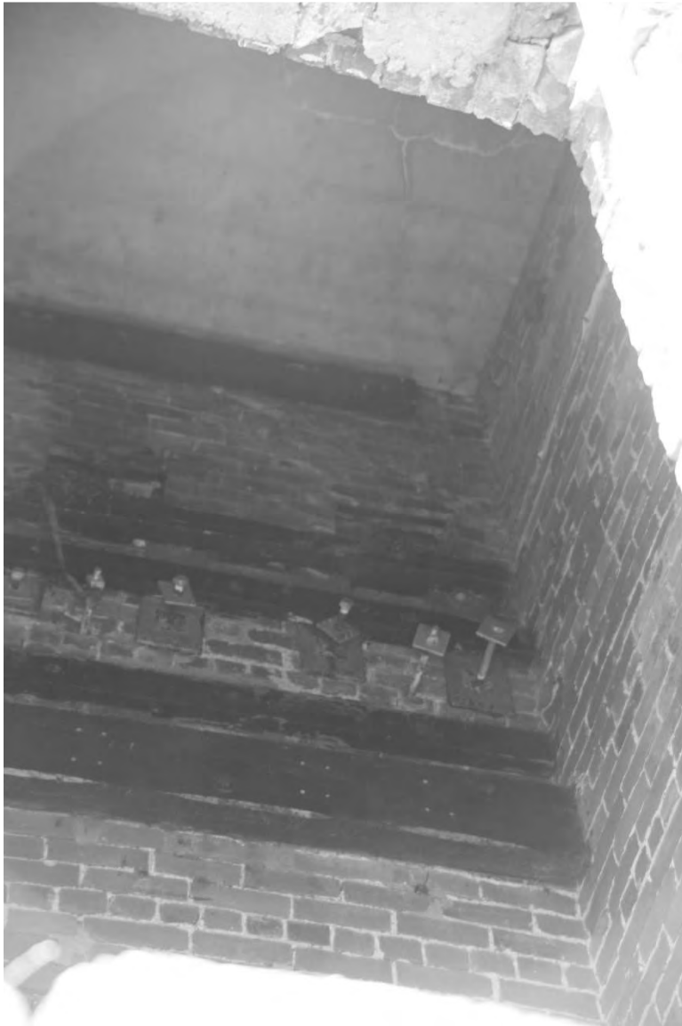
Photo 9) Durham Cable House, interior walls and ceiling
