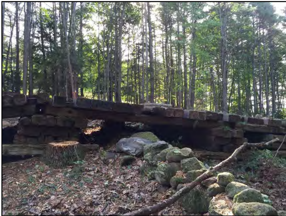
Figure 1. Timber Matting Over Stone Wall Segment
