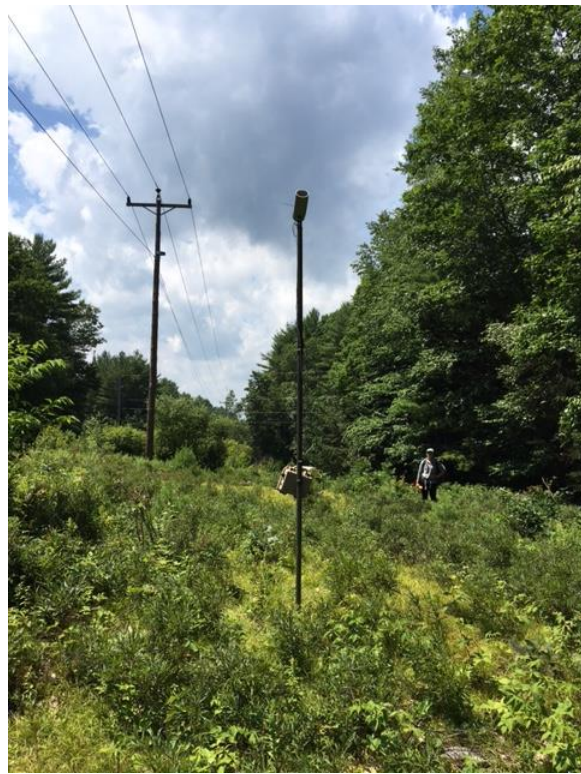
Figure C-66. Segment 11 – facing west.
