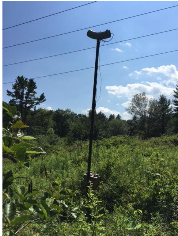
Figure C-60. Segment 10 – facing west.
