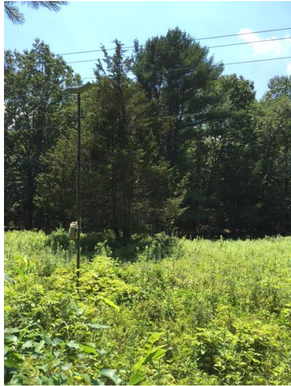
Figure C-54. Segment 9 – facing west.
