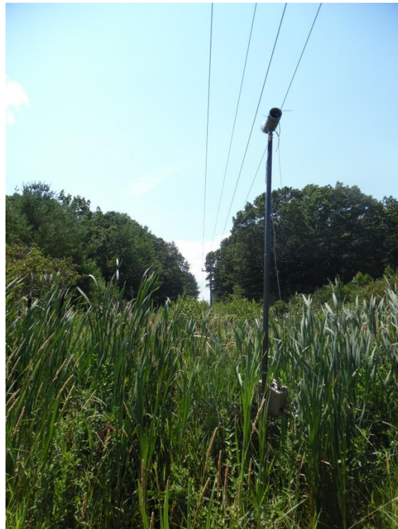
Figure C-36. Segment 6 – facing west.
