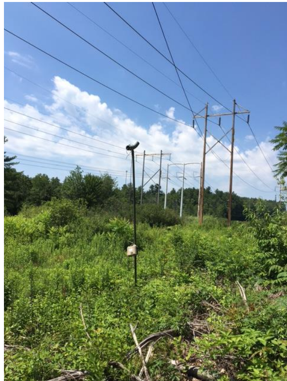
Figure C-120. Segment 20 – facing west.
