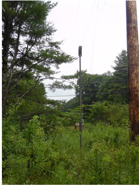
Figure C-78. Segment 13 – facing west.
