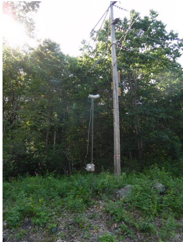
Figure C-96. Segment 16 – facing west.
