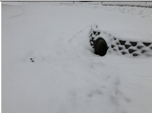
29 Gundalow - 1 (Drainage Area)
