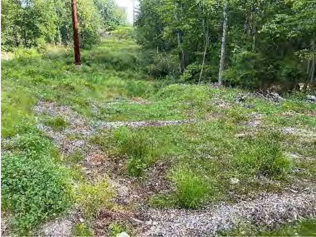
Fig 1: Lower portion of slope between Strs. 28 and 29. Viewing northeast. (08-17-21)
