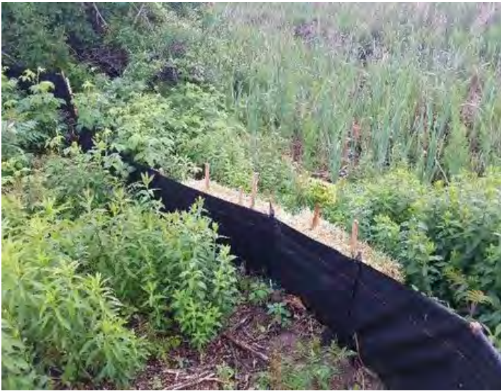
Fig 5: Silt fence installed between Str. 137 and wetland NW37. Viewing north. (6-14-19).
