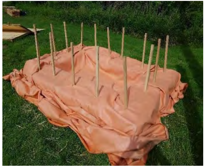
Fig 6: The dewatering apparatus next to Colovos Rd. Waiting for materials to finish the install. Viewing east. (6-14-19).
