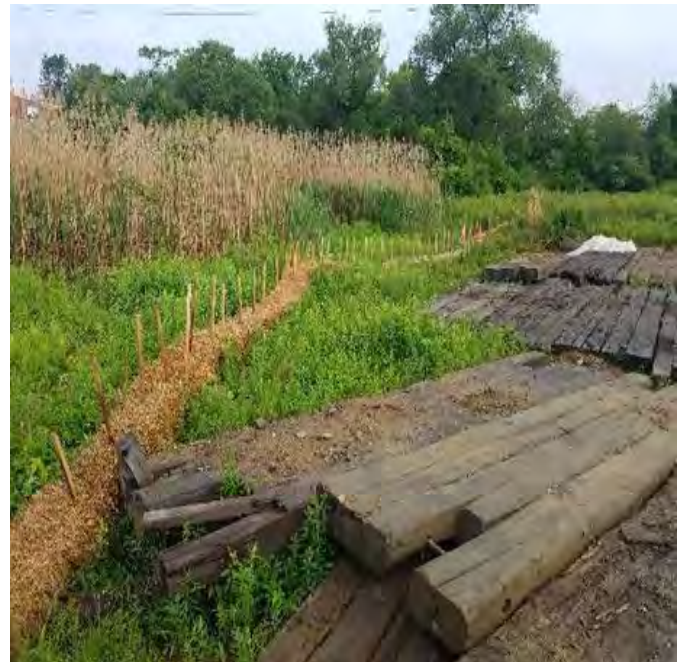
Fig 4: Straw bales installed between Str. 138 and Wetland NW37. Viewing north. (6-14-19).
