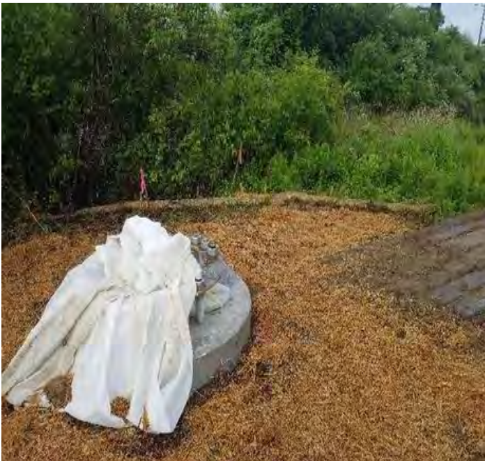
Fig 3: Straw waddles installed between Str. 139 and Wetland NW37. Viewing southeast. (6-14-19).
