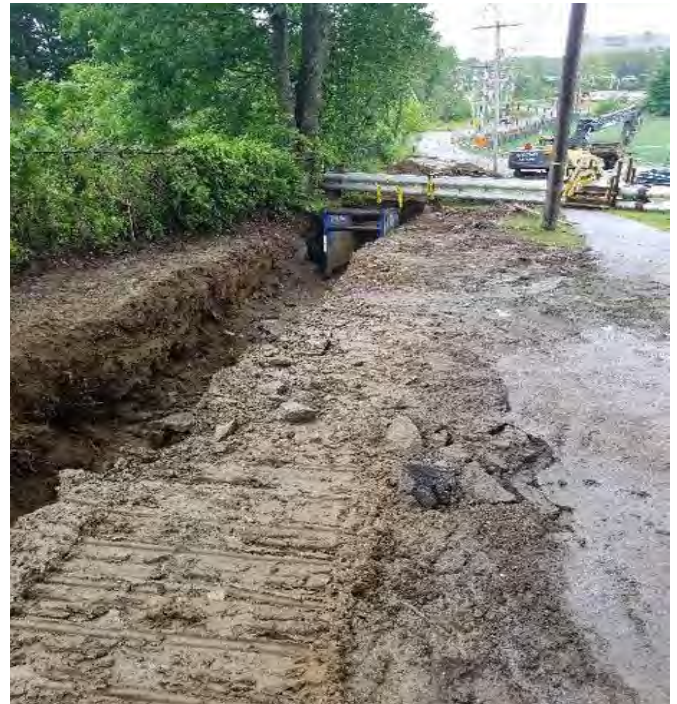
Fig 4: Trenching for duct bank next to field house at UNH. Viewing south. (6-21-19).
