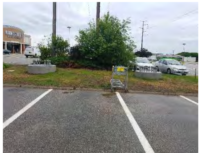
Fig 14: Str. F107-135 foundation in Newington mall parking lot, note germination. Viewing northeast. (6-21-19).
