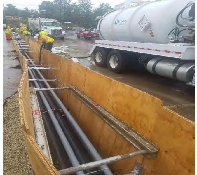
Fig 2: Vac truck is used to pump rain water out of trench in "A" lot. Viewing south. (6-20-19).
