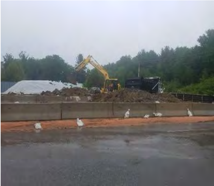
Fig 1: GZA continues to haul out soil from stockpile area in "A" lot. Viewing north. (6-20-19).
