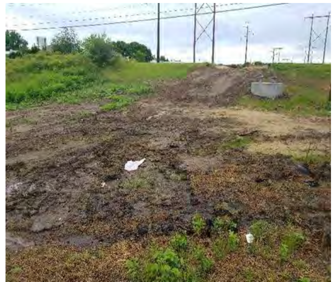
Fig 12: Exposed soil next to Str. F107-136 due to utility work along Woodbury Ave. Viewing southwest. (6-21-19).
