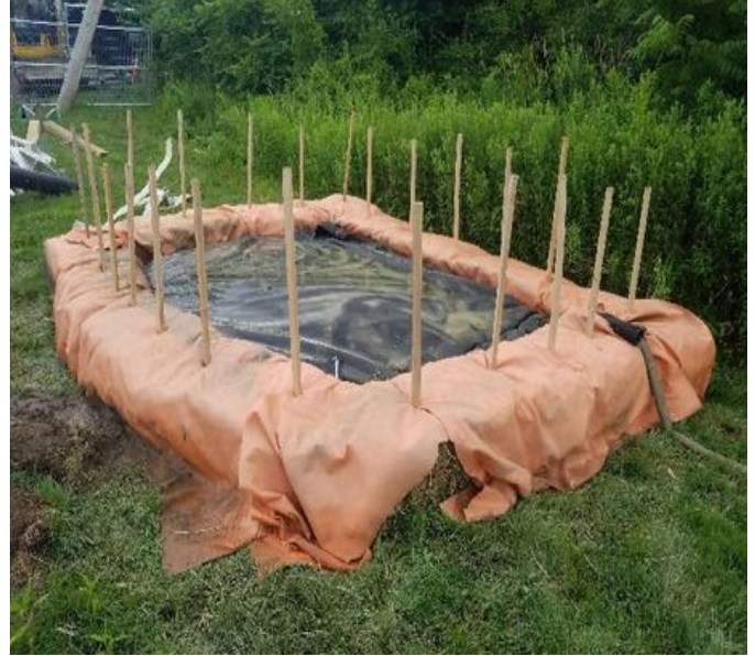
Fig 2: McCourt built a larger dewatering apparatus with new filters. Viewing north. (7-12-19).
