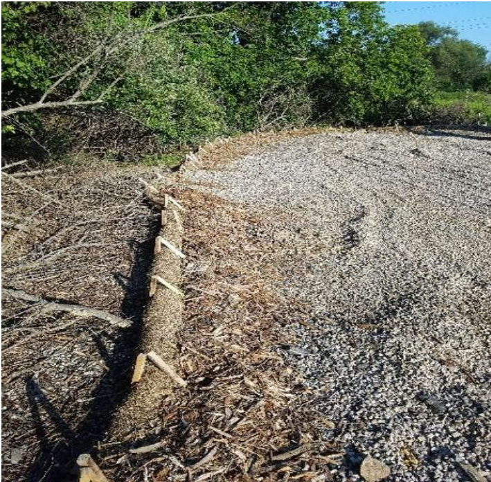
Fig 3: Combined berm installed in the laydown yard off of Gosling Rd. Viewing east. (7-14-19).
