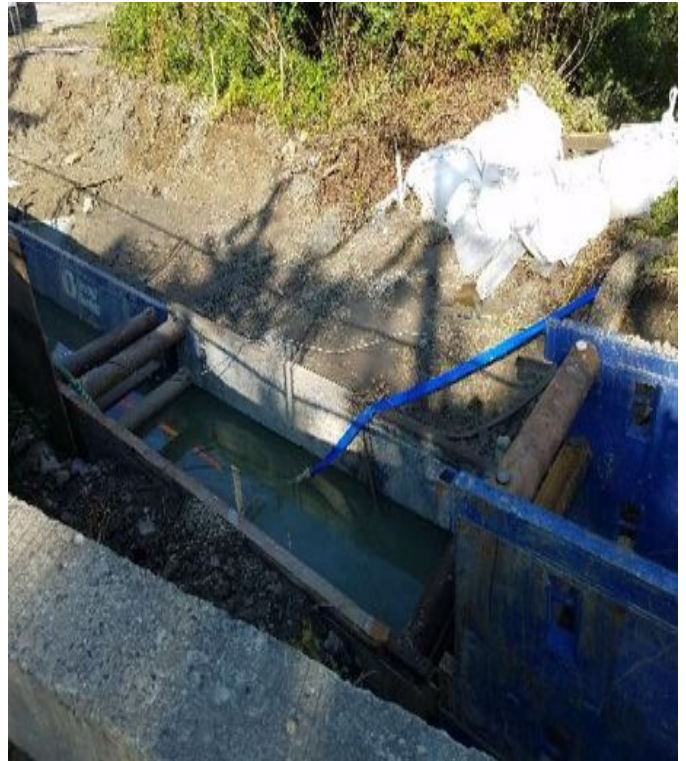
Fig 8: Trenching activities through College Brook. Viewing west. (7-14-19).
