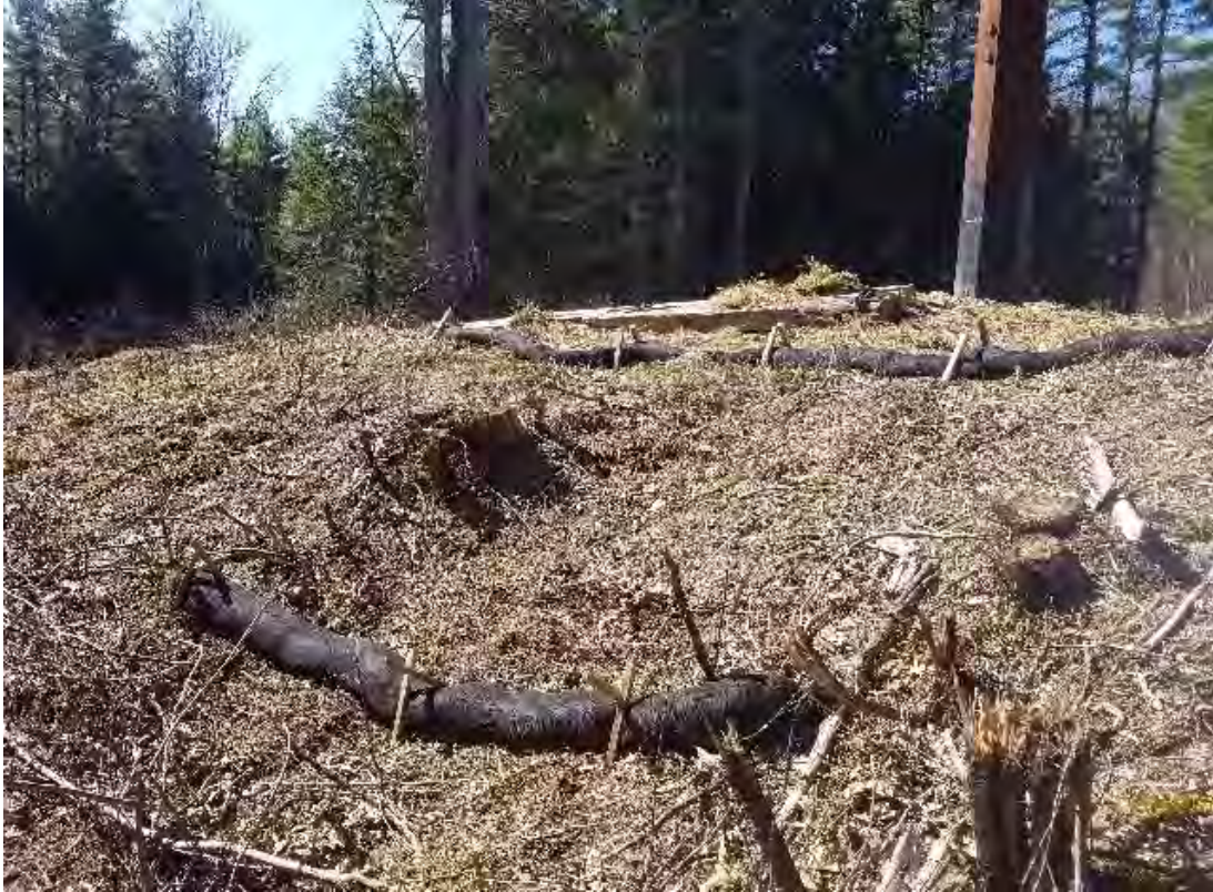
Fig 9: Additional filter sock installed in swale downslope of Str. 51. Viewing southwest. (04-07-20).
