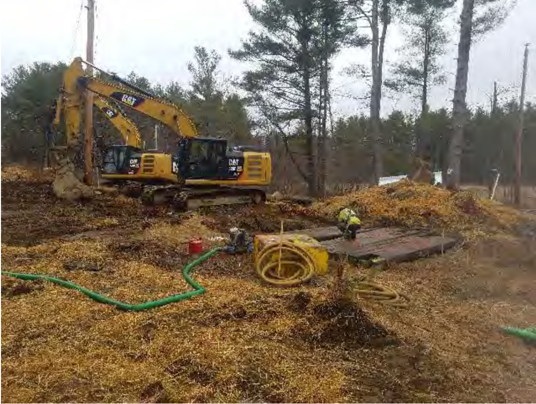
Fig 3: Excavating foundation for Str. 94. Viewing northwest. (04-02-20).
