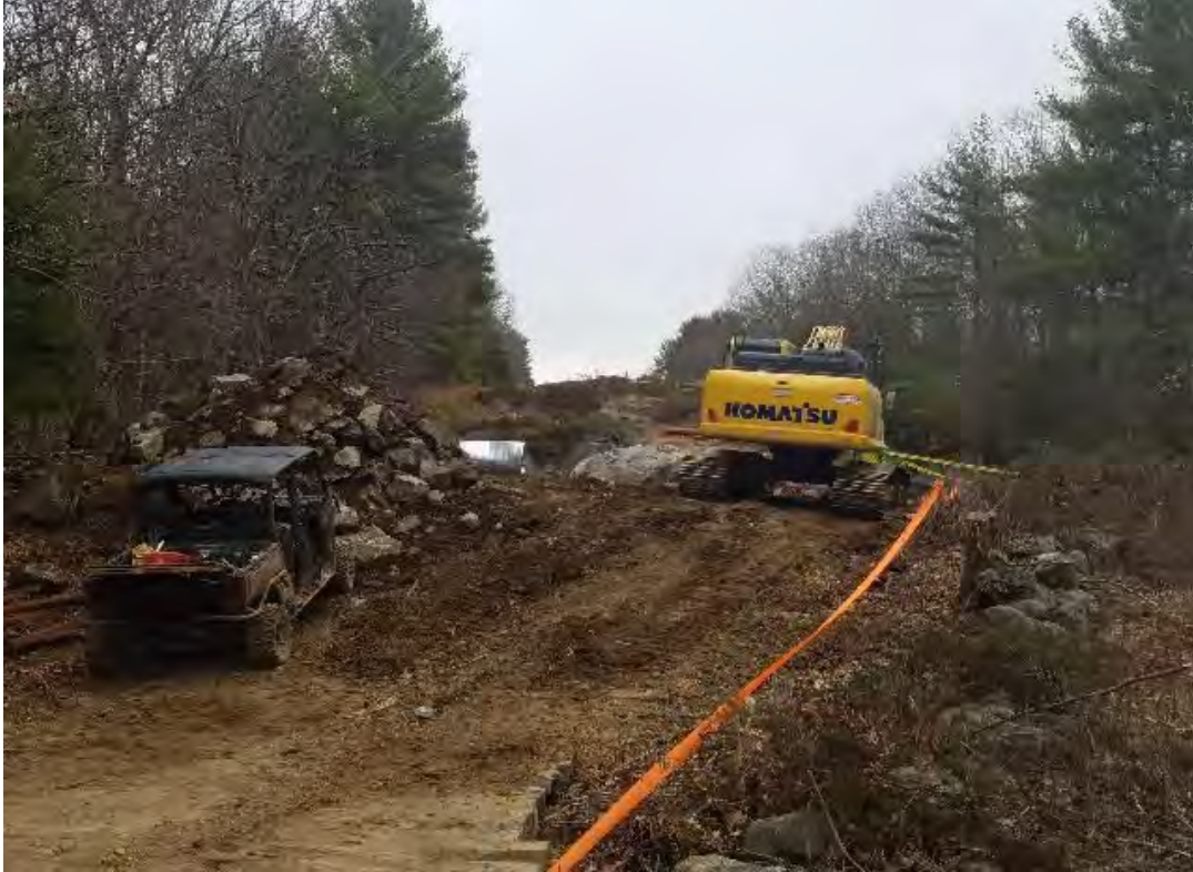
Fig 11: Crew continues to hammer ledge at Str. 79. Viewing southeast. (04-08-20).
