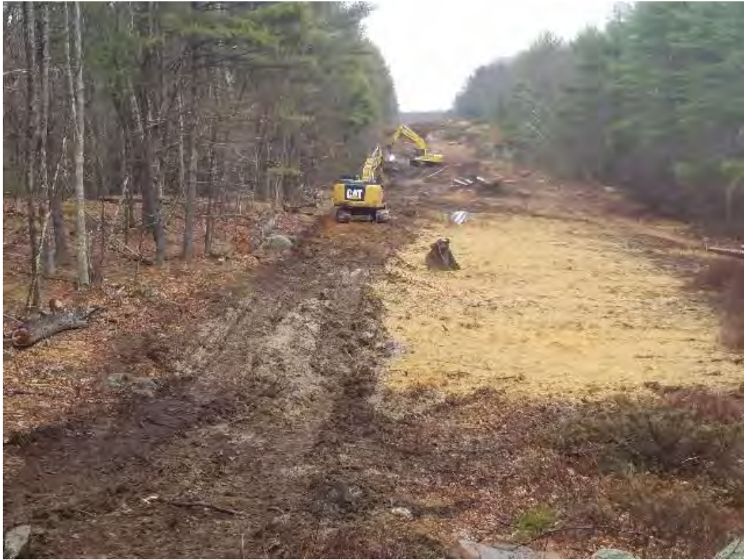
Fig 1: Restoring upland access road next to Str. 78 work area. Viewing east. (04-02-20).
