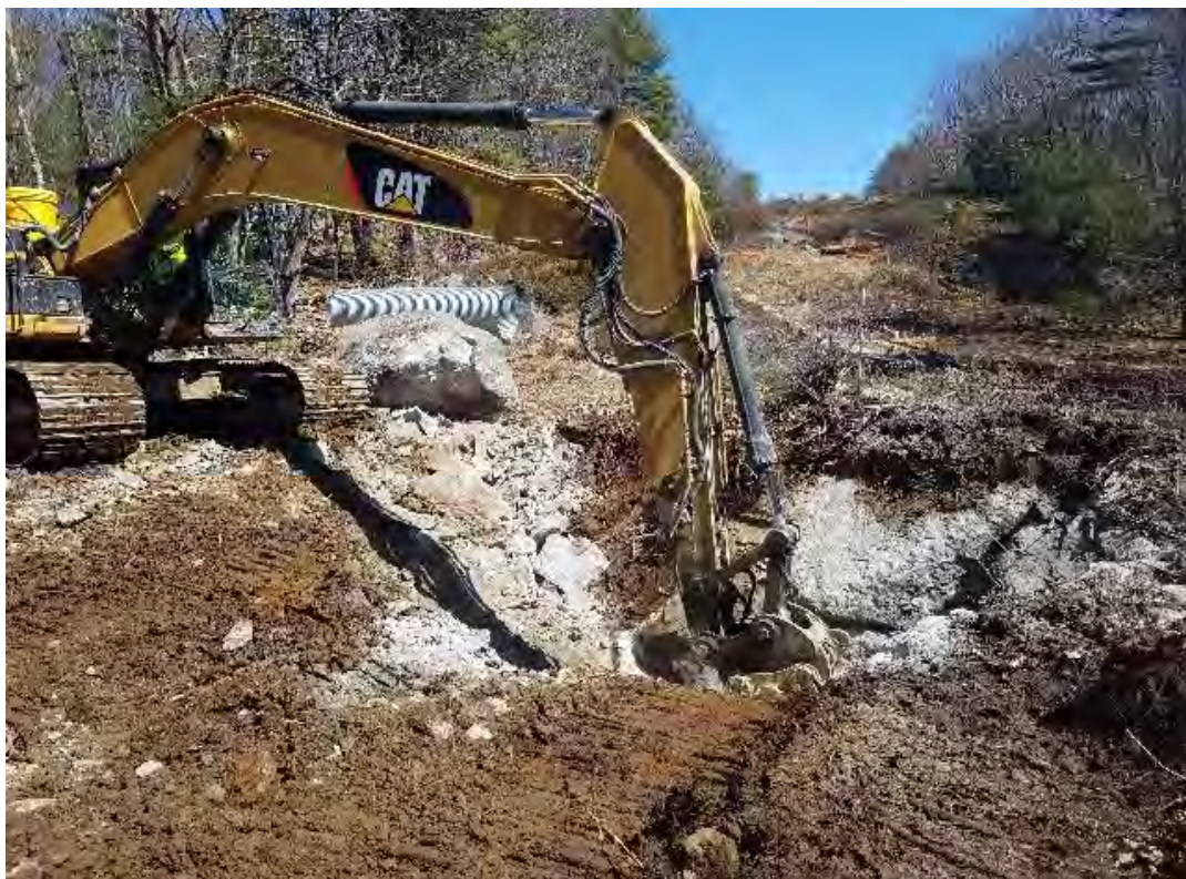
Fig 6: Hammering ledge at Str. 79. Viewing east. (04-06-20).
