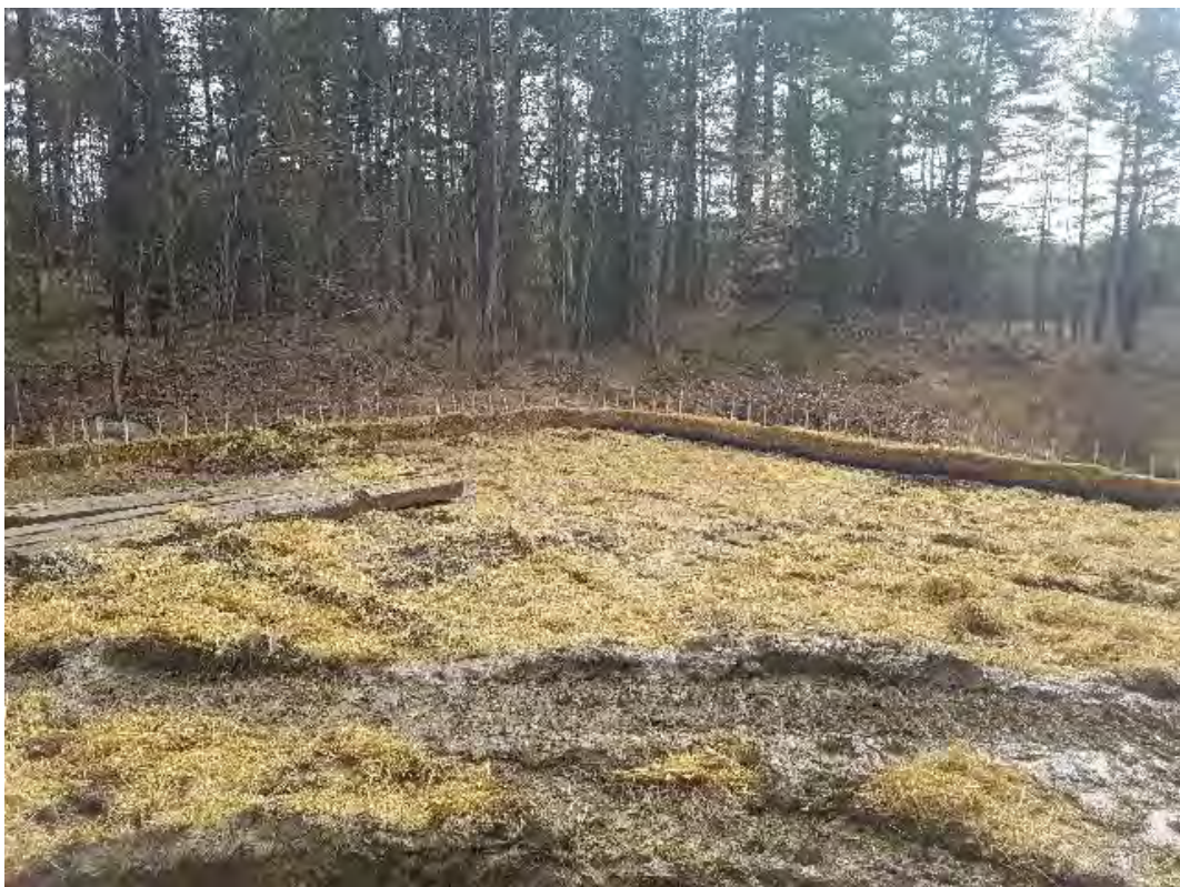
Fig 4: Str. 93 foundation can set and work area. Viewing east. (04-10-20).
