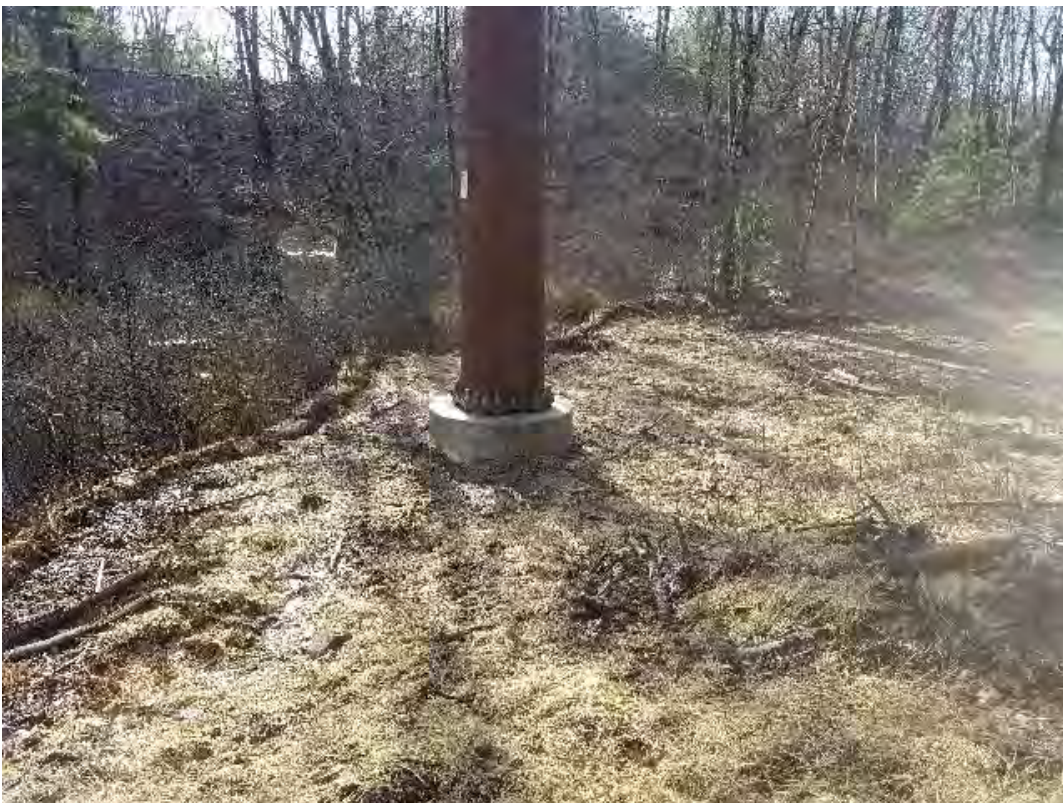
Fig 2: Str. 28 foundation. Viewing east. (04-10-20).
