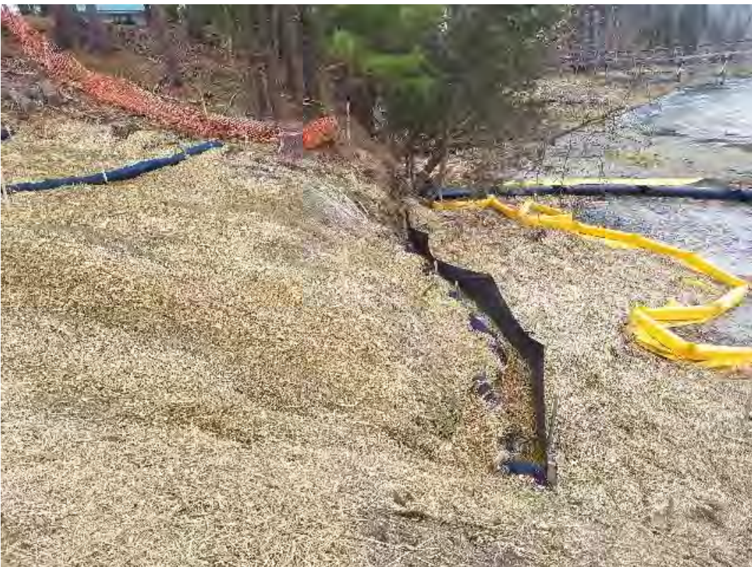
Fig 10: BMPs at toe of slope, east side of the Bay. Note marine wrack trapped behind silt curtain. Straw is stable on slope. Viewing south. (04-10-20).
