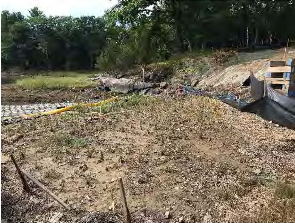
Fig 9: Salt marsh restoration at Eversource property/west side of the bay. Viewing south. (08-19-20).
