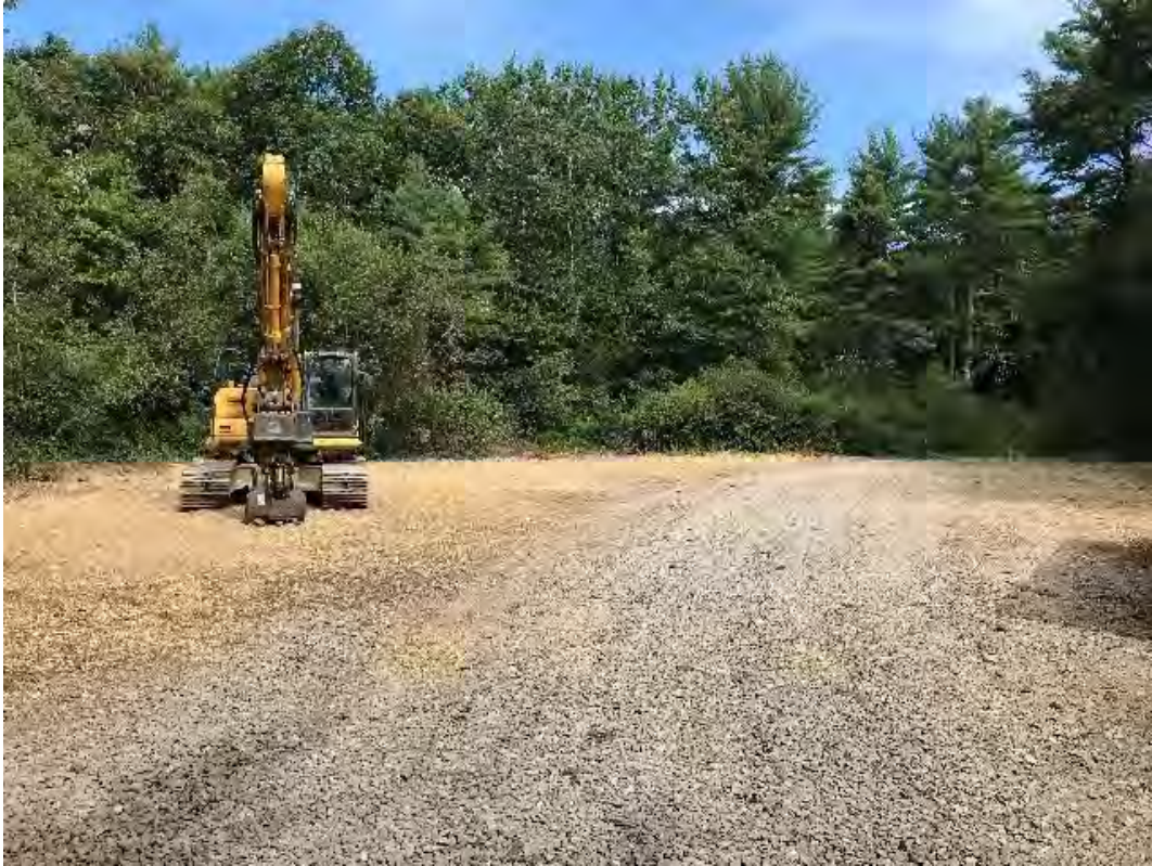
Fig 1: Bennett Rd. staging area. Gravel path restored and exposed soil seeded and mulched. Viewing north. (08-19-20).
