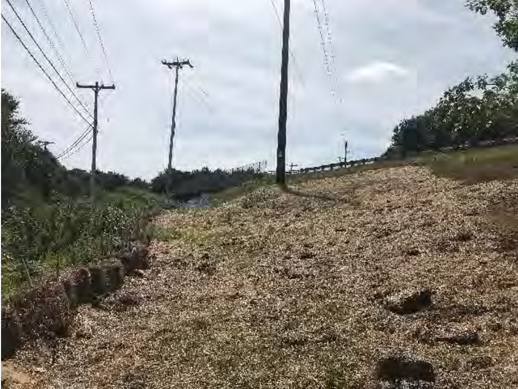
Fig 3: Str. 6 work area is revegetating, but straw bales shall remain in place for now. Viewing southwest. (09-01-20).
