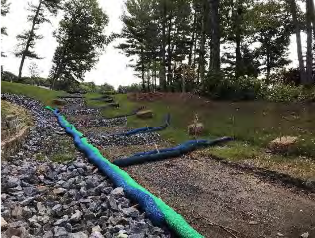
Fig 1: Slope above the manhole at Gundalow Landing/east side of the bay. Viewing east. (09-14-20)
