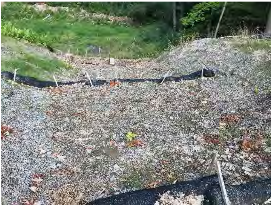
Fig 10: Swale between Strs. 28 and 29 remains stable. Viewing north. (09-11-20)
