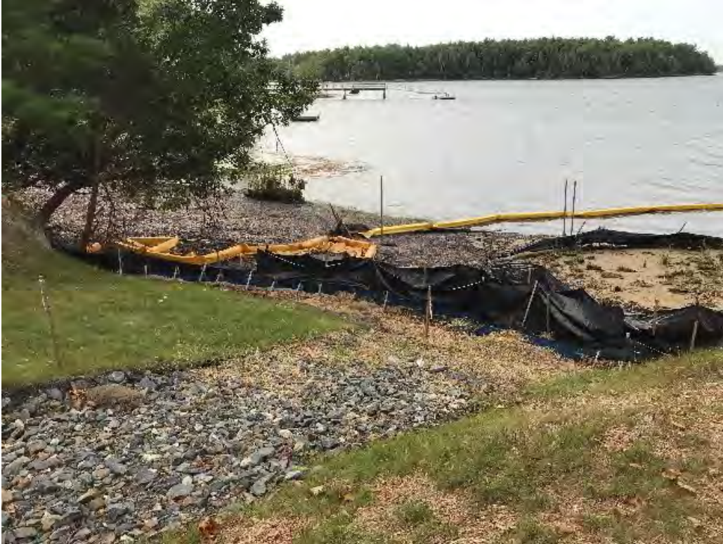
Fig 3: Toe of the slope below the manhole at Gundalow Landing/east side of the bay. Viewing south. (09-14-20)
