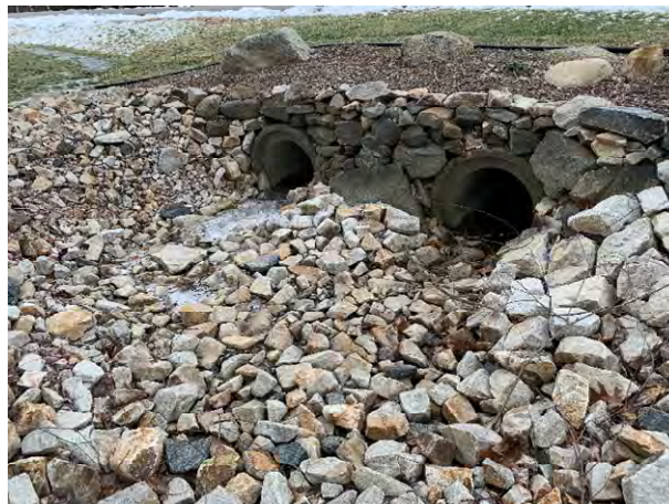
64 Gundalow - 2 (Drainage Course)
