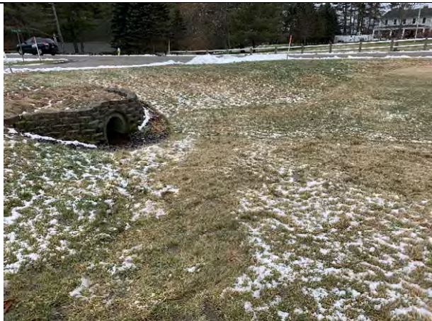
29 Gundalow - 1 (Drainage Area)
