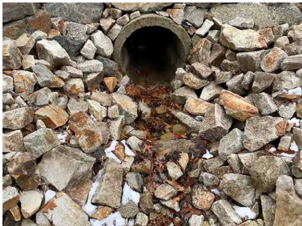
64 Gundalow - 1 (Drainage Course)
