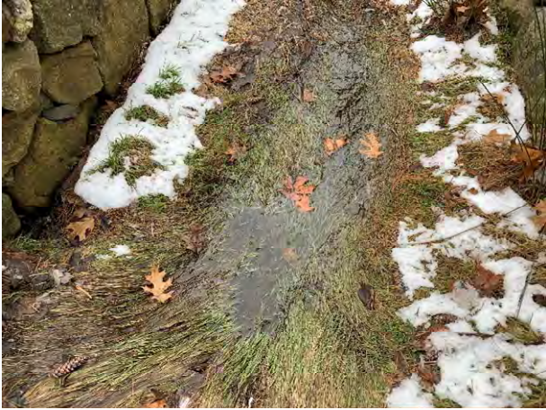
4 Brickyard Circle – 3 (Drainage Course)
