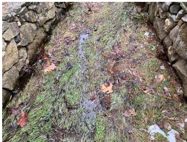
4 Brickyard Circle - 2 (Drainage Course)
