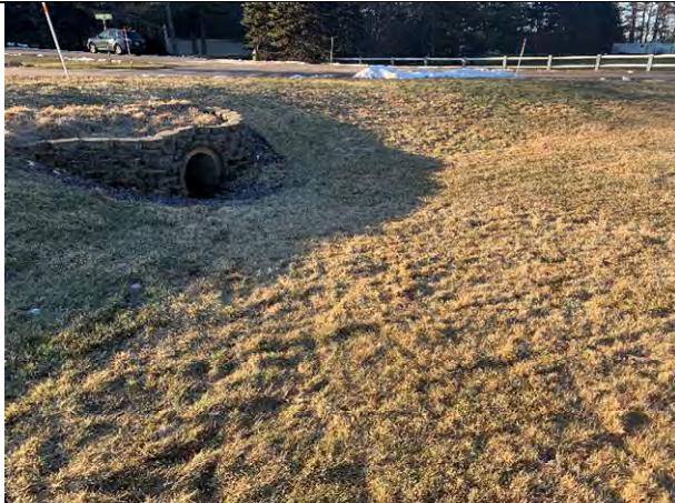
29 Gundalow - 1 (Drainage Area)
