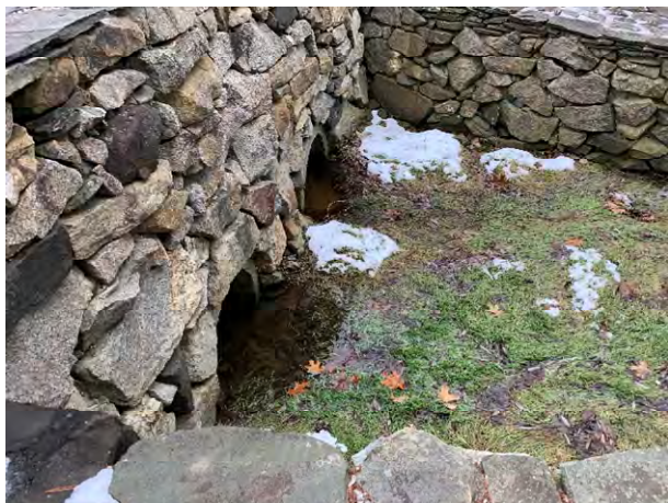
4 Brickyard Circle - 1 (Drainage Course)
