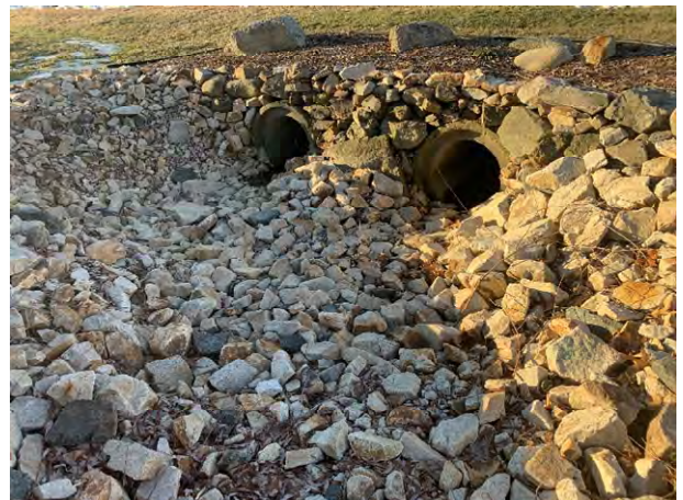
64 Gundalow - 2 (Drainage Course)
