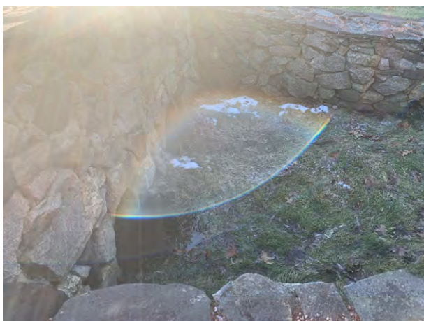
4 Brickyard Circle - 1 (Drainage Course)
