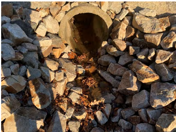
64 Gundalow - 1 (Drainage Course)
