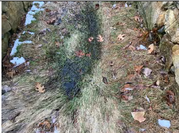
4 Brickyard Circle – 3 (Drainage Course)
