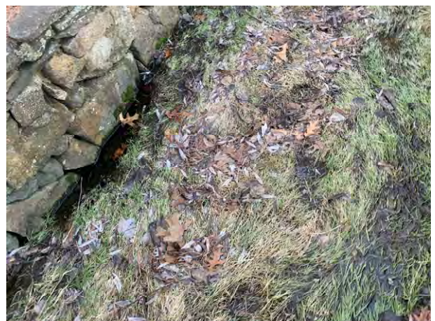
4 Brickyard Circle - 2 (Drainage Course)
