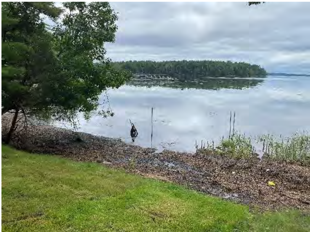
Fig 10: Toe of slope at Gundalow Landing/east side of the bay. Viewing south. (08-20-21)
