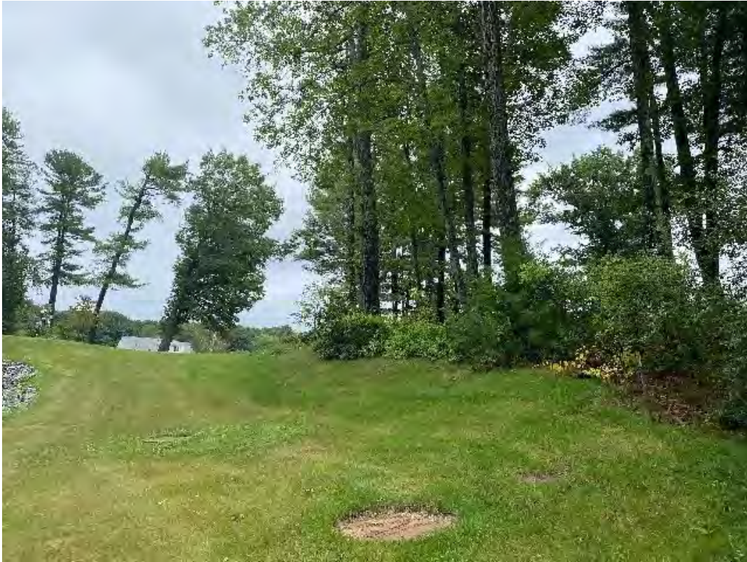
Fig 9: Slope above the manhole at Gundalow Landing/east side of the bay. Viewing east. (08-20-21)
