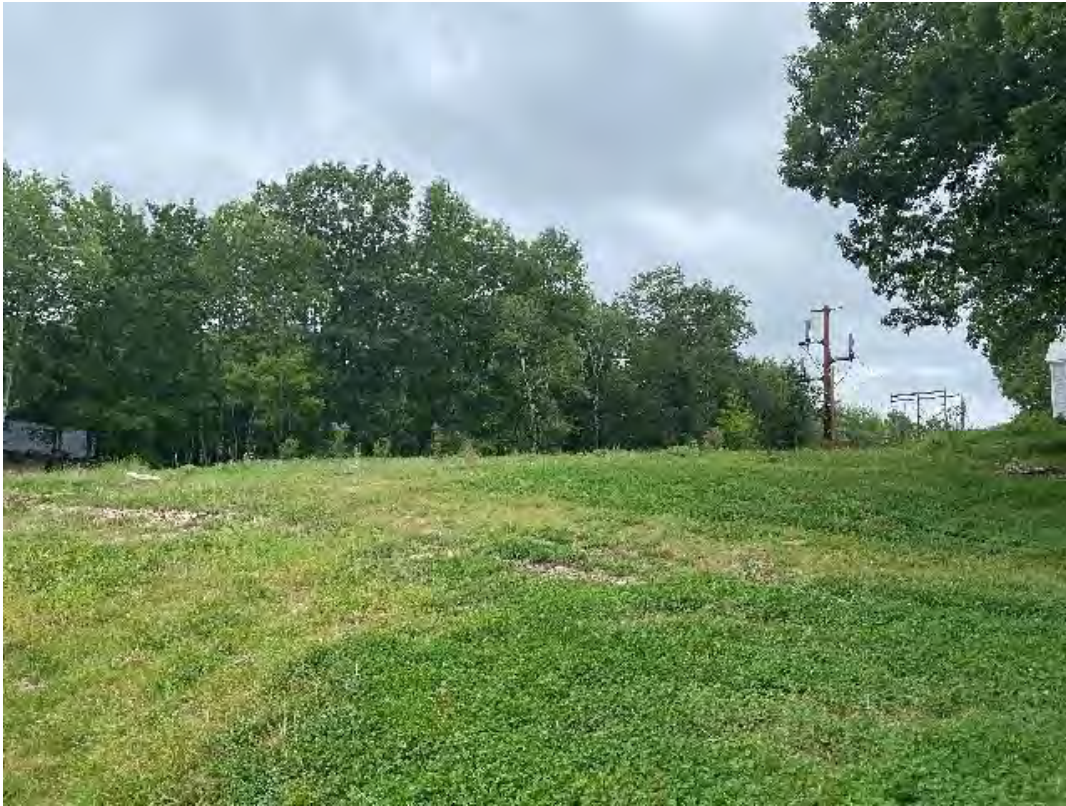
Fig 3: Slope above the cable house at the west side of the bay. Viewing southwest. (08-20-21)
