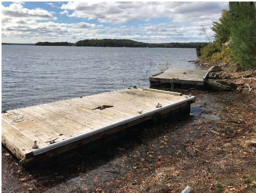
Floating docks positioned on top of the salt marsh restoration at Gundalow Landing/east side of the bay. Viewing north. (10-18-21)
