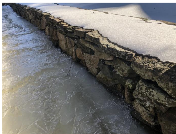
4 Brickyard Circle - 2 (Drainage Course)
