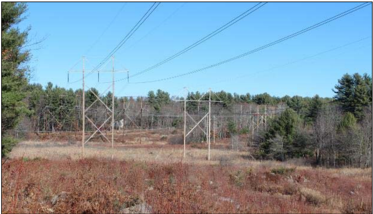
Photo Inset 8. Viewpoint 109, Musquash Conservation Area, view to the northeast from Landing Trail toward existing ROW.
