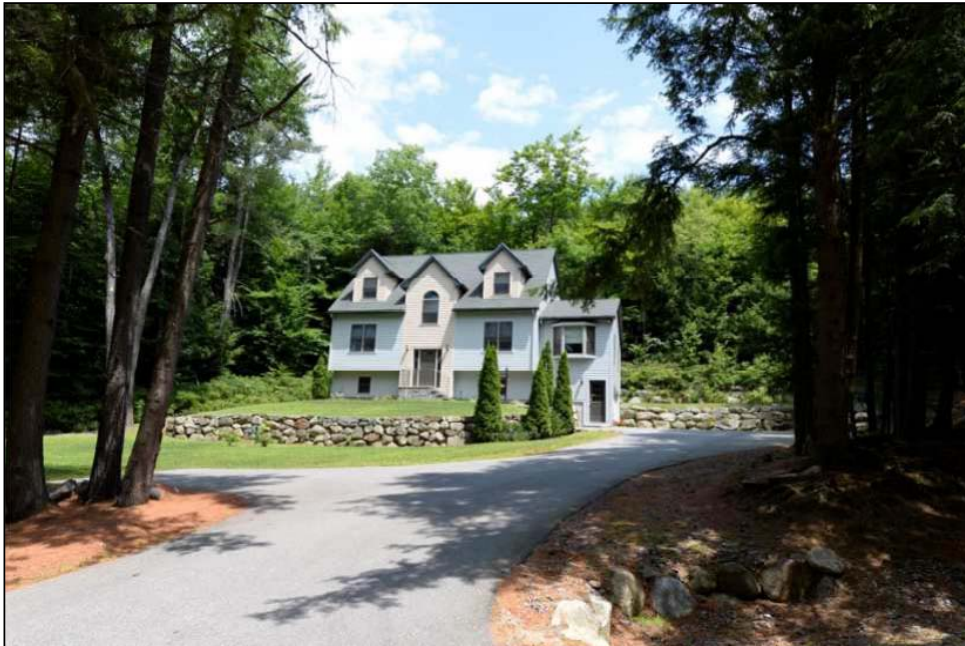
Figure 5.2.6.4 Photograph of Lot 71 (non-abutting) as Improved (taken 7/14/2014)
