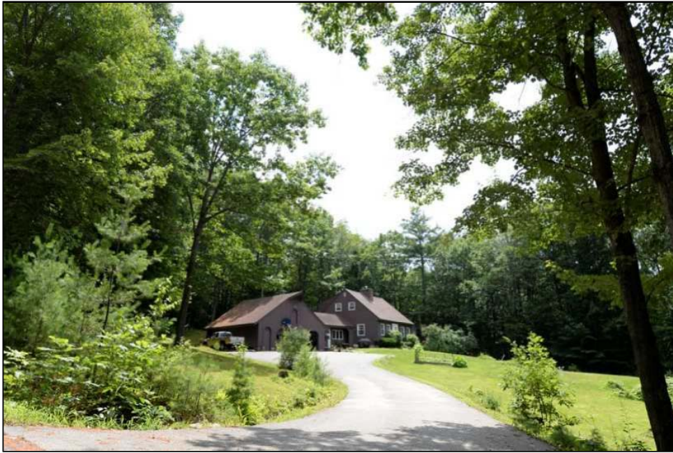
Figure 5.2.6.3 Photograph of Lot 48 (non-abutting) as Improved (taken 7/14/2014)
