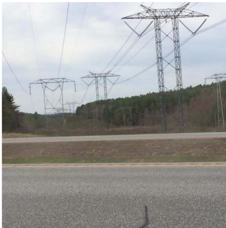
Figure 4.1.1 Photograph of Corridor #1 Cross Section
