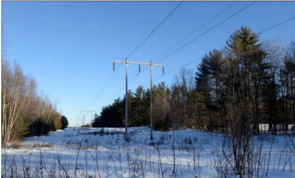
Figure 4.1.2 Photograph of Corridor #2 cross section
