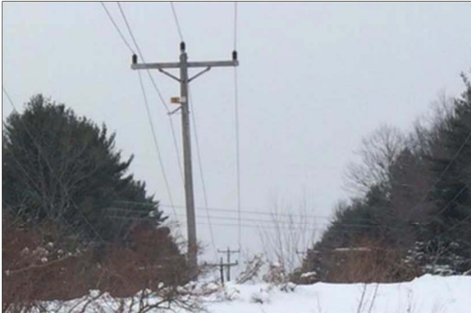
Figure 4.1.5 Photograph of Study Area #3 -- 34.5 kV Cross Section
