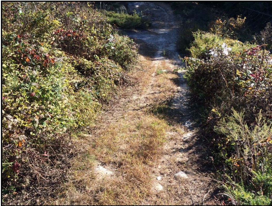
Photo 44: View north of NEP access road through WA 62 where timber access matting and stone ford installation is planned. 10/09/2014.
