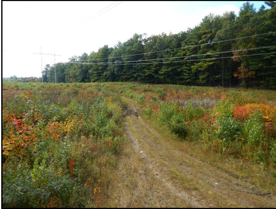
Photo 119: View west toward Eversource access road crossing WA 146A where timber access matting is planned. Tree clearing also planned within this wetland. 09/26/2014.
