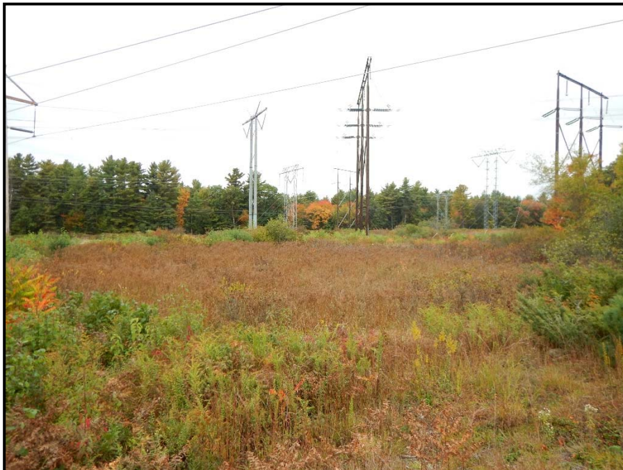
Photo 86: View west toward WA 108. Construction work pad to extend into edge of wetland as part of a large pull pad site. Guy anchor installation also proposed within this wetland. 10/02/2014.
