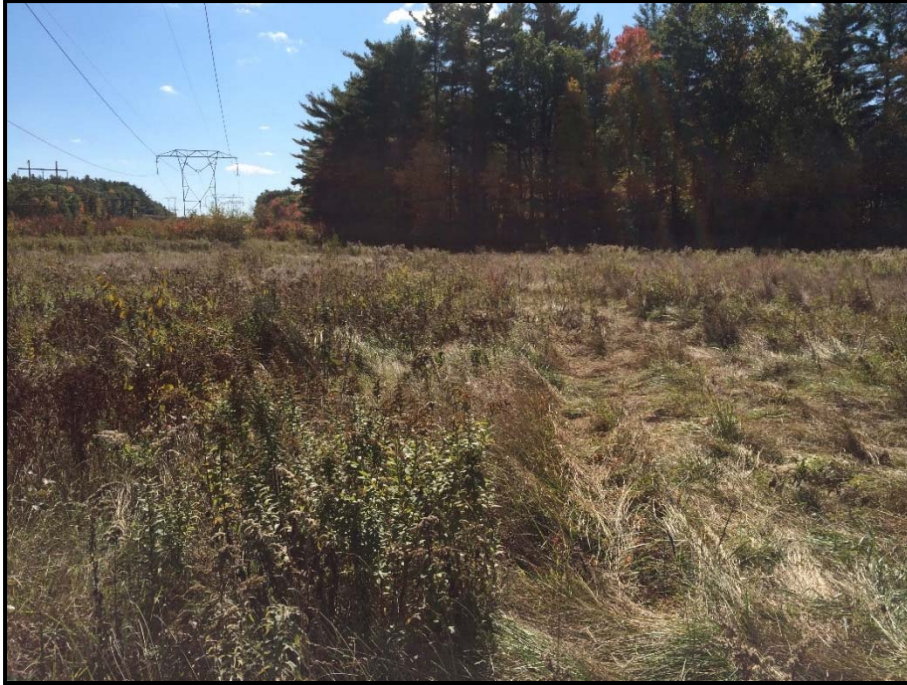
Photo 37: View southeast toward WA 54A. Two construction work pads planned near this area, one for pole installation outside wetland and one to install Structure 51 within wetland. Timber access matting planned along NEP access road into wetland. 10/09/2014.
