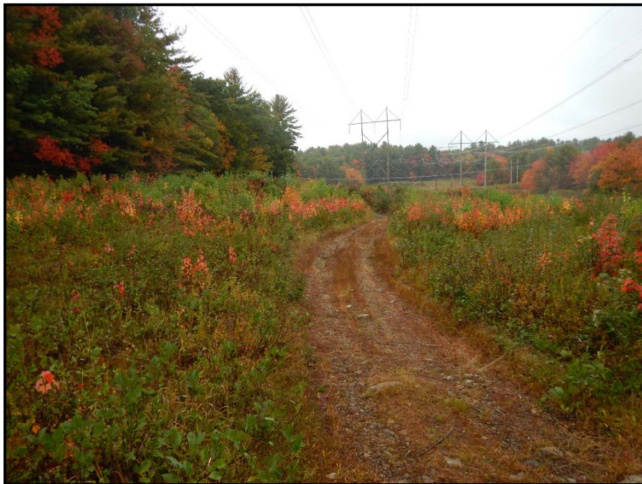
Photo 104: View north of Eversource access road through WA 127 where timber access matting is planned. 10/01/2014.
