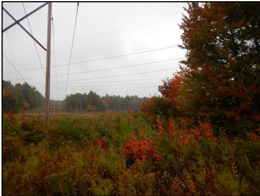
Photo 106: View west toward WA 128. Planned location of a large construction work pad area for pull pad and guard protection area. Structure 253 proposed to be installed just inside this wetland. Tree clearing proposed to right of photo. Guy anchor installation also proposed in this area. 09/30/2014.
