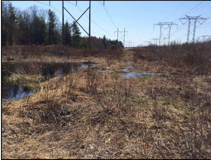
Photo 19: View southeast of access road where timber access matting is planned across Nesenkeag Brook (SA-32). Limited tree clearing is planned along the eastern edge of the ROW (photo left). 4/22/2015.
