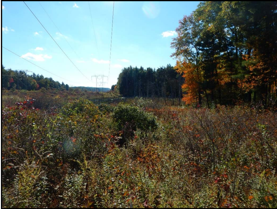
Photo 51: View south toward WA 75A. Construction work pad planned to extend into wetland for pole installation outside of wetland. 10/08/2014.
