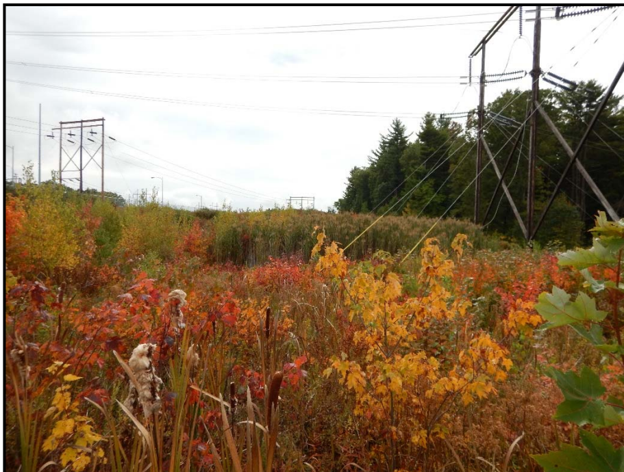
Photo 134: View south toward WA 167 near the Scobie Pond Substation. A construction work pad is to be placed over part of this wetland for a pull pad site. 09/24/2014.
