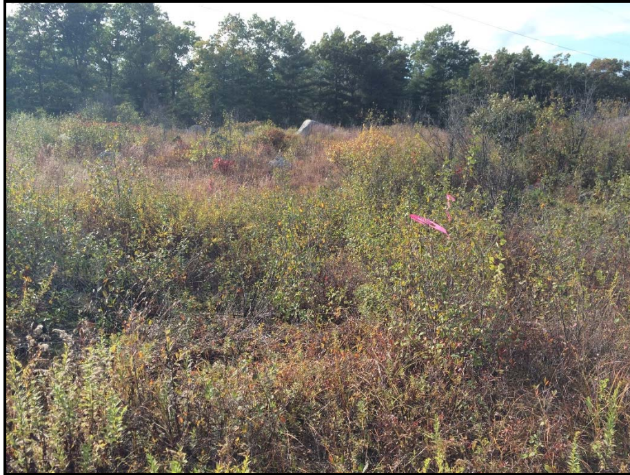
Photo 5: View west toward WA 34. Construction work pad is planned in this area for pole installation and removal outside of wetland. 10/07/2014.
