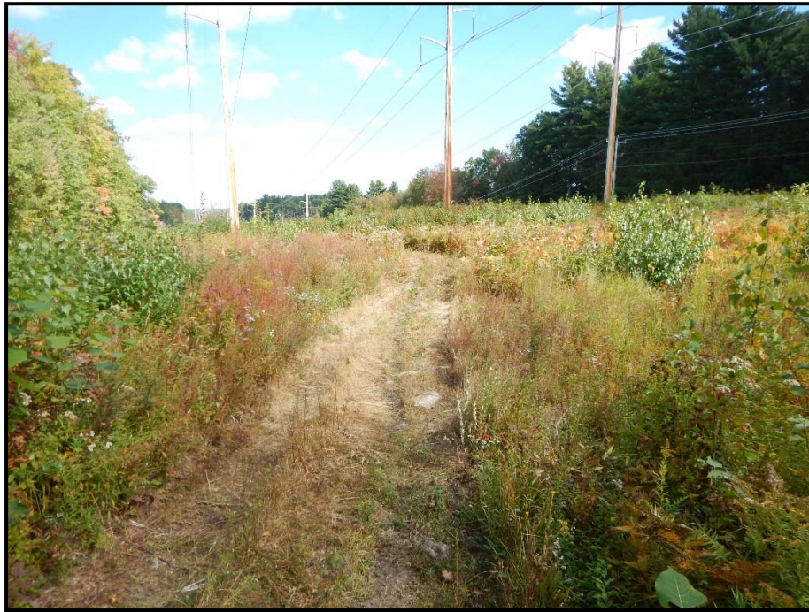
Photo 121: View southeast of WA 147. Timber access matting planned where Eversource access road crosses wetland. 09/26/2014.
