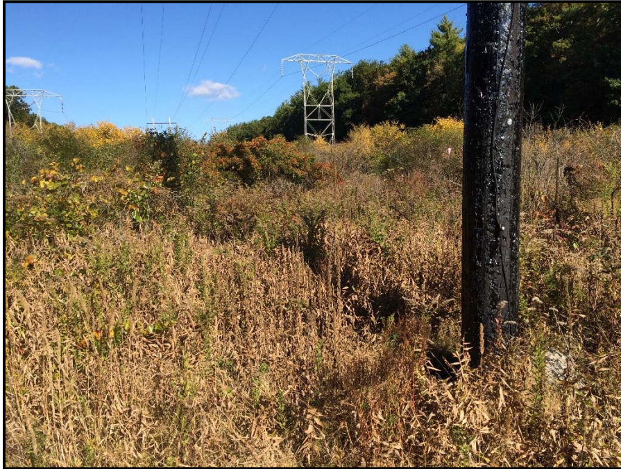
Photo 29: View north of WA 50 where construction work pad is planned for pole installation and removal outside of wetland. General location of proposed permanent road crossing. 10/09/2014.
