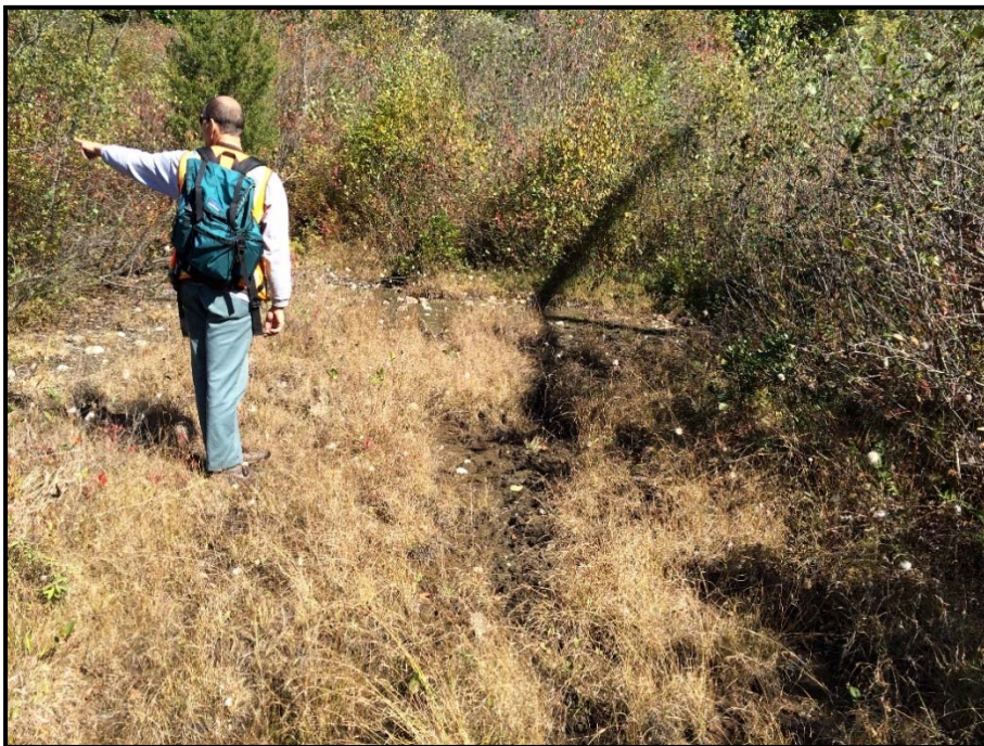
Photo 38: View west toward WA 59. Construction work pad for pole installation and removal outside of wetland planned in this area. 10/09/2014.
