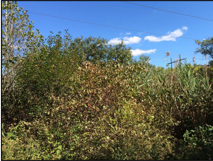
Photo 39: View east toward WA 59. Construction work pad for pole installation and removal outside of wetland planned in this section of the wetland. Timber access matting also planned along NEP access road along edge of wetland. 10/09/2014.
