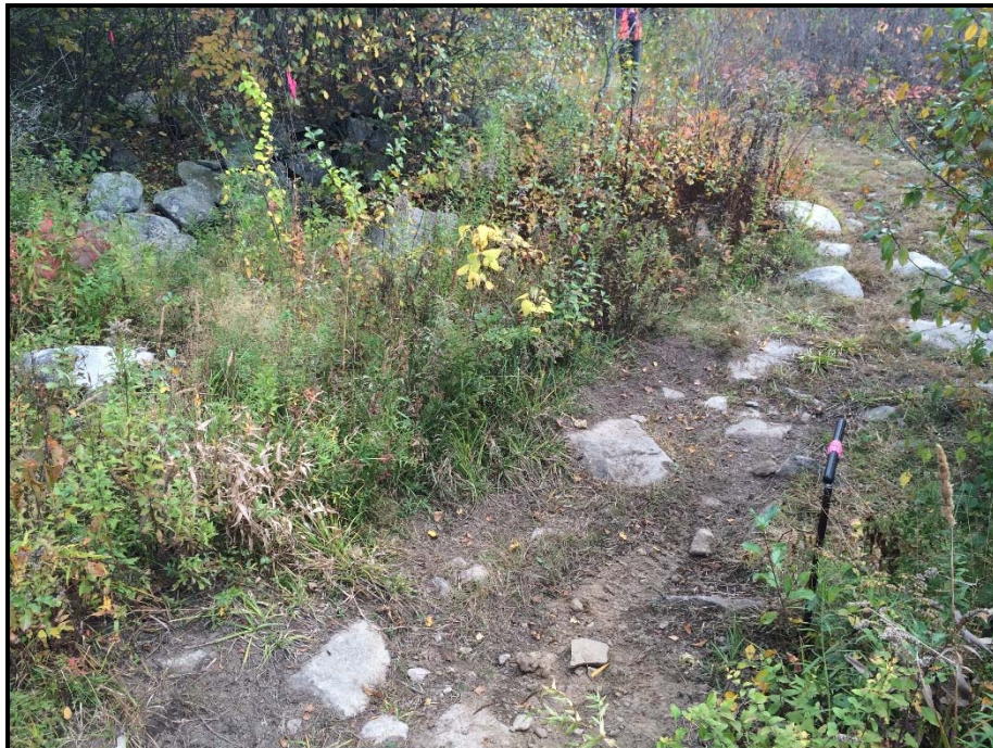
Photo 10: View southeast of access road through WA 37 where timber access matting is planned. Construction work pad for pole installation is planned just outside of wetland. 10/08/2014.
