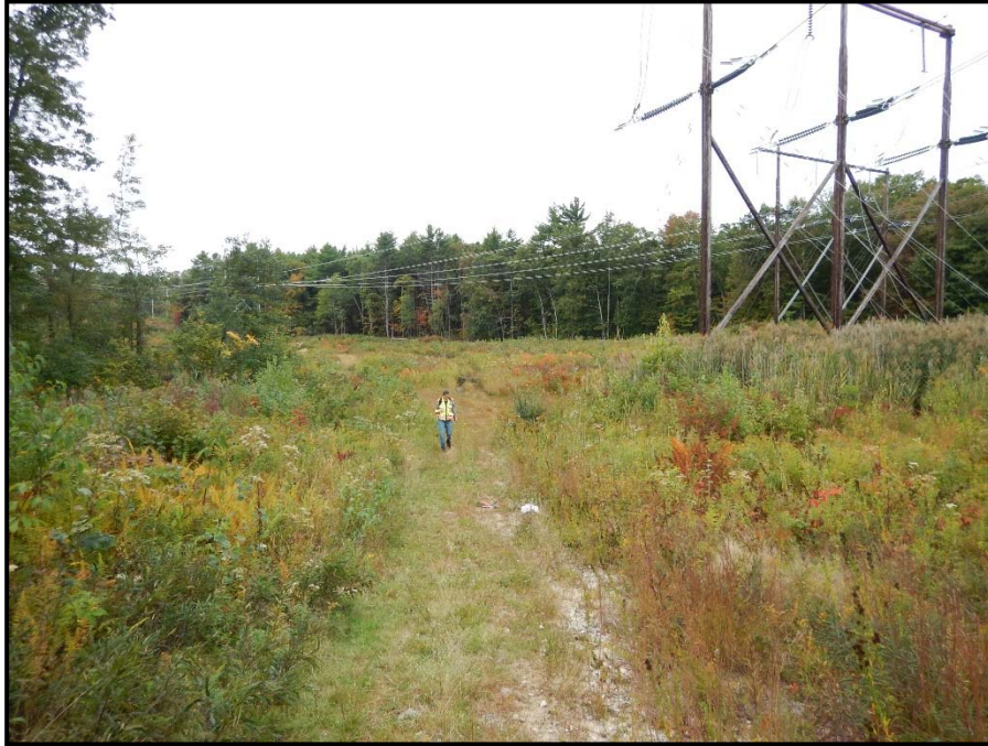
Photo 133: View southwest of Eversource access road next to WA 166. A construction work pad is to be placed over part of this wetland for a pull pad site. General location for guy wire installation. 09/24/2014.
