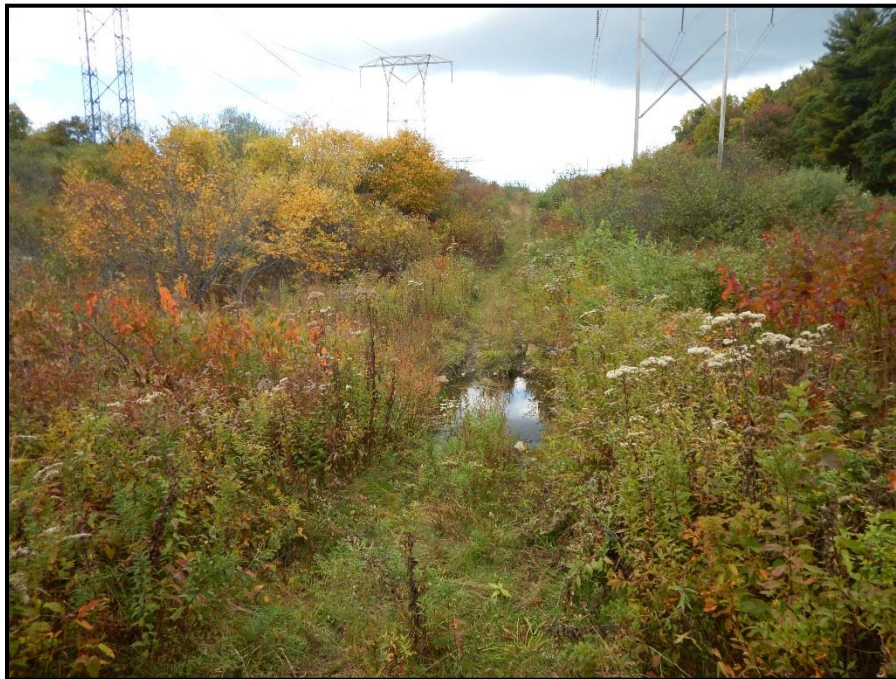
Photo 56: View west of Eversource access road through WA 77C where timber access matting is planned. Tree clearing planned within wetland along edge of ROW. 10/08/2014.
