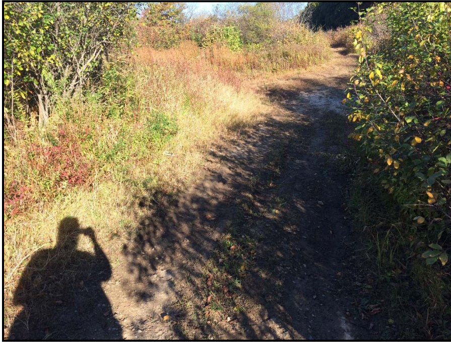
Photo 25: View north of access road through WA 48 where timber access matting is planned. Construction work pad also planned in this general area for pole installation and removal outside of wetland. 10/09/2014.
