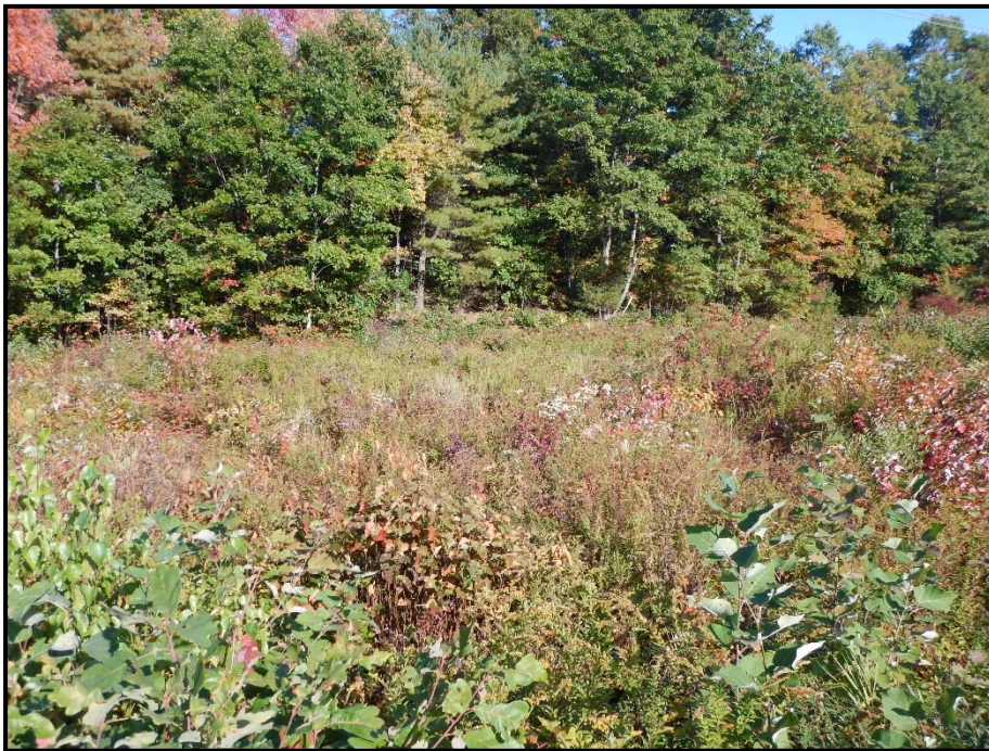
Photo 70: View east toward WA 95. Construction work pad for pole installation to extend into wetland area. Pole to be installed just outside of wetland. 10/03/2014.
