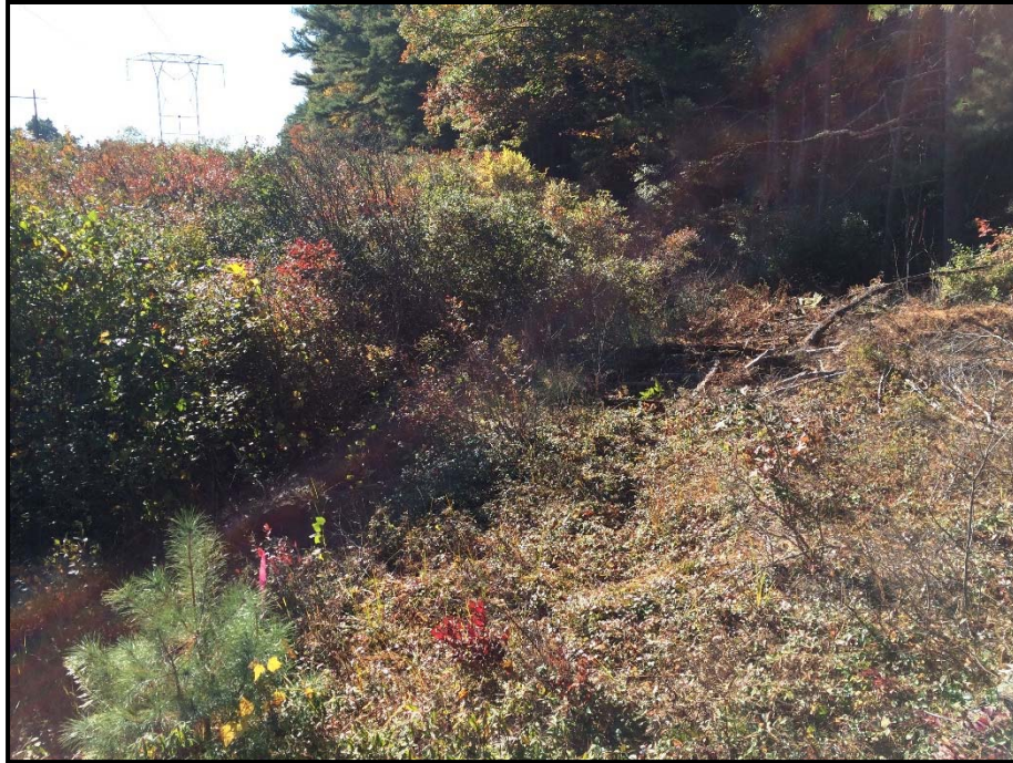
Photo 27: View southeast toward WA 49 where a construction work pad is planned to extend into a section of the wetland for pole installation outside of wetland. 10/09/2014.
