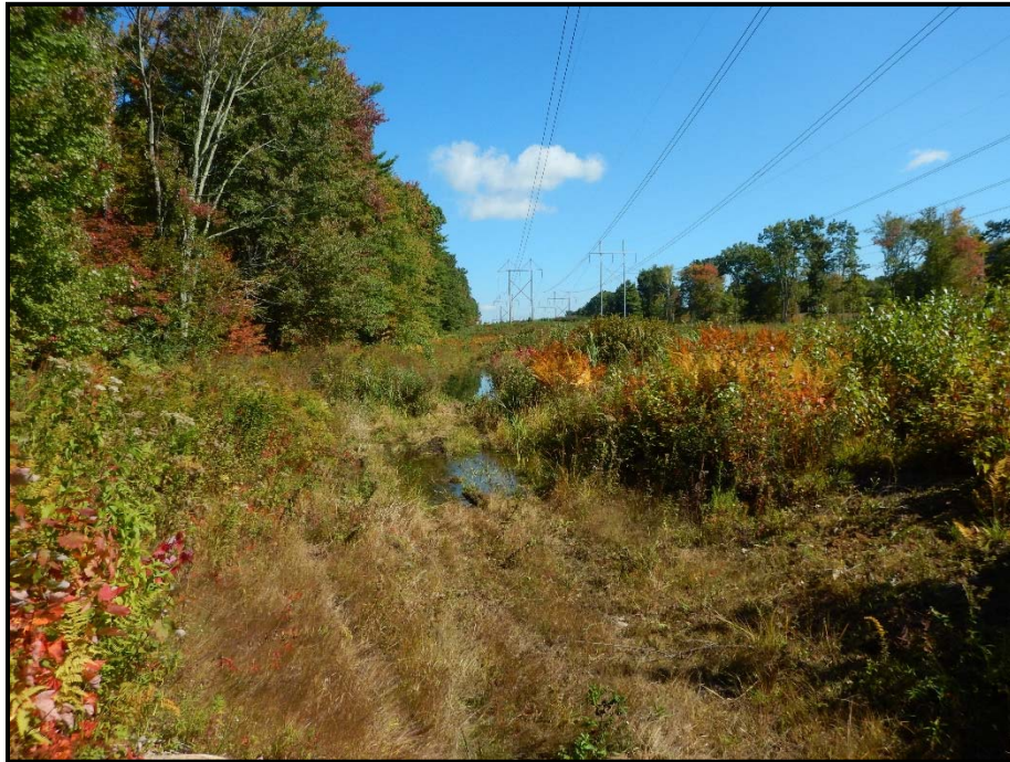
Photo 124: View northeast along Eversource access road toward WA 149A where timber access matting is planned. Construction work pad for pole installation and guard protection area proposed east of photo. Tree clearing also planned within this wetland. 09/25/2014.
