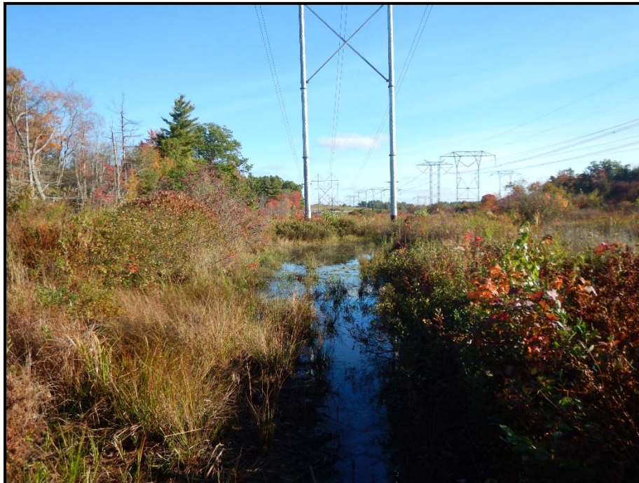
Photo 68: View east of WA 93. Timber access matting is planned along access road through the wetland (to left of photo). Further southeast of photo a construction work pad is planned to install Structure 222 within the wetland. Tree clearing planned to the left of photo. 10/03/2014.
