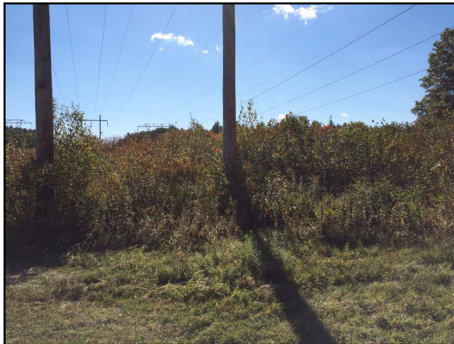
Photo 36: View south toward WA 54. A construction work pad for pole installation will extend into the wetland to the left of photo. Tree clearing proposed in wetland along edge of ROW. 10/09/2014.
