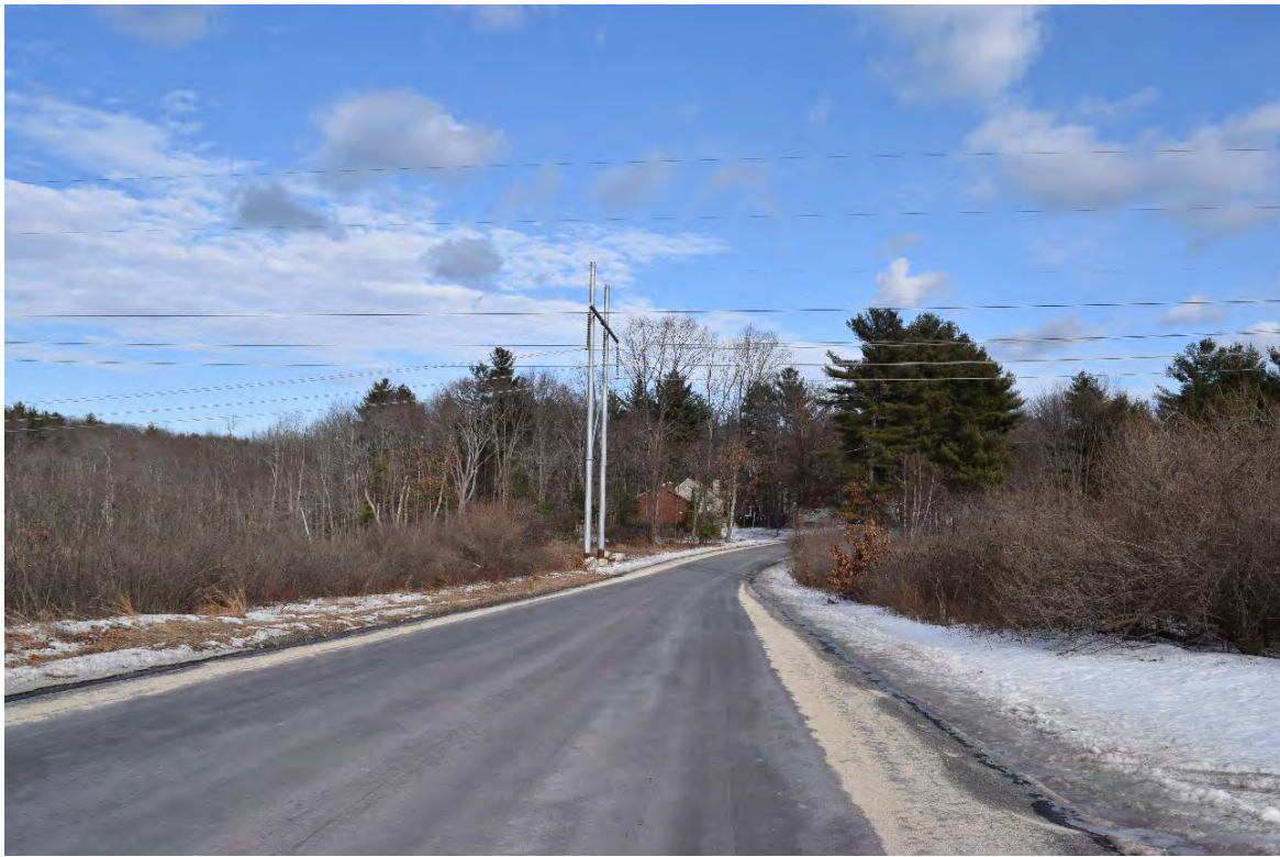
Photograph 20. Looking northeast up David Drive.
