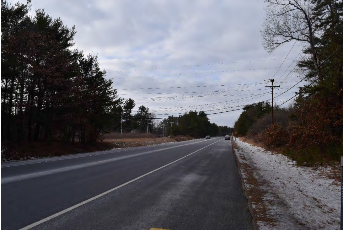
Photograph 3. Looking southwest up Bridge Street.
