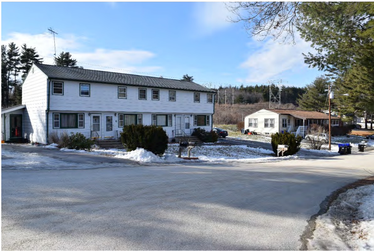
Photograph 16. Looking northwest from the intersection of Bockes Road and Hopkins Drive.
