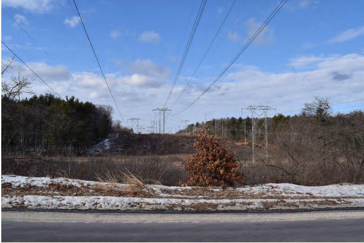
Photograph 19. Looking northwest at Project Area.
