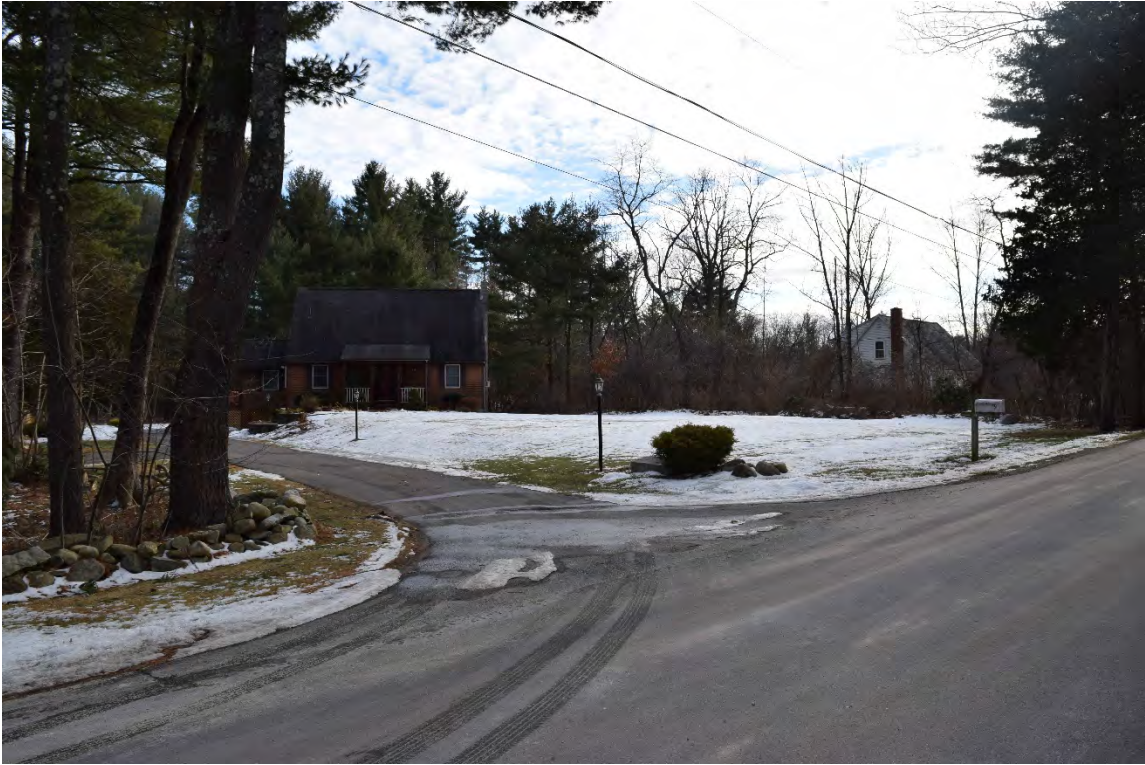
Photograph 26. Looking southwest at 9 Dan Hill Road.
