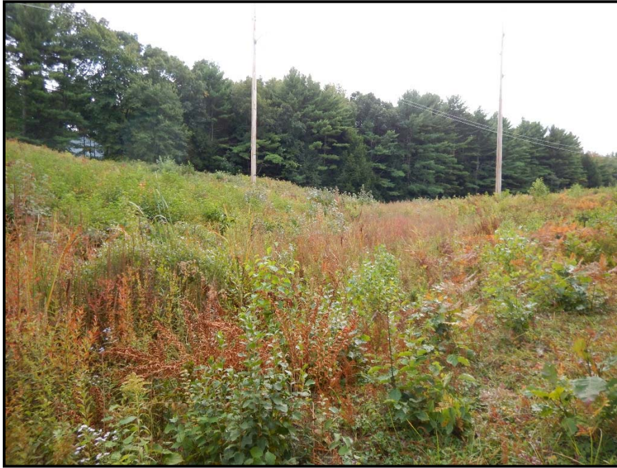
Photo 129: View east toward southern end of WA 160 along access road. Access matting is planned to the east. Tree clearing planned to right of photo. To the north of photo is the proposed location for a construction work pad for pole installation. 09/25/2014.
