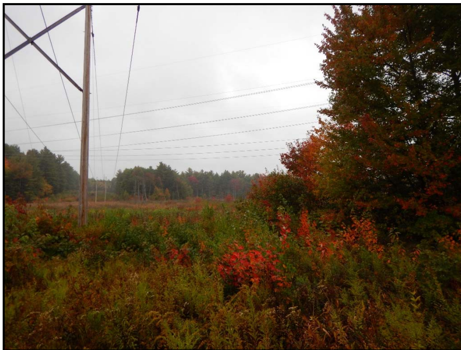
Photo 106: View west toward WA 128. Planned location of a large construction work pad area for pull pad and guard protection area. Structure 253 proposed to be installed just inside this wetland. Tree clearing proposed to right of photo. Guy anchor installation also proposed in this area. 09/30/2014.
