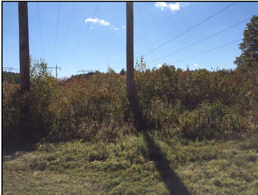
Photo 36: View south toward WA 54. A construction work pad for pole installation will extend into the wetland to the left of photo. Tree clearing proposed in wetland along edge of ROW. 10/09/2014.
