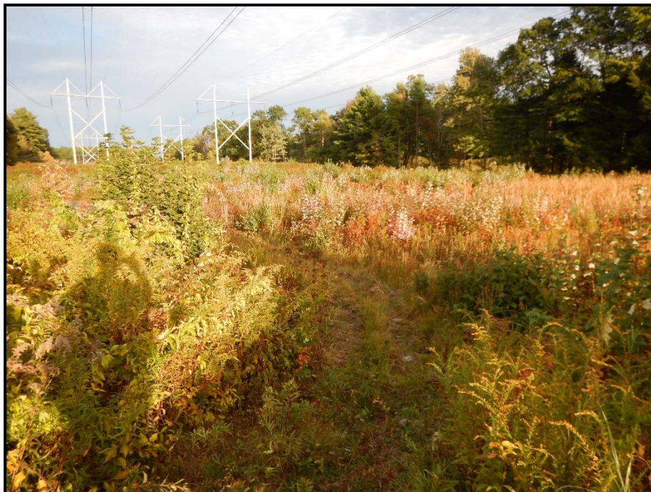
Photo 128: View east toward Eversource access road through WA 156 where timber access matting is planned. 09/25/2014.
