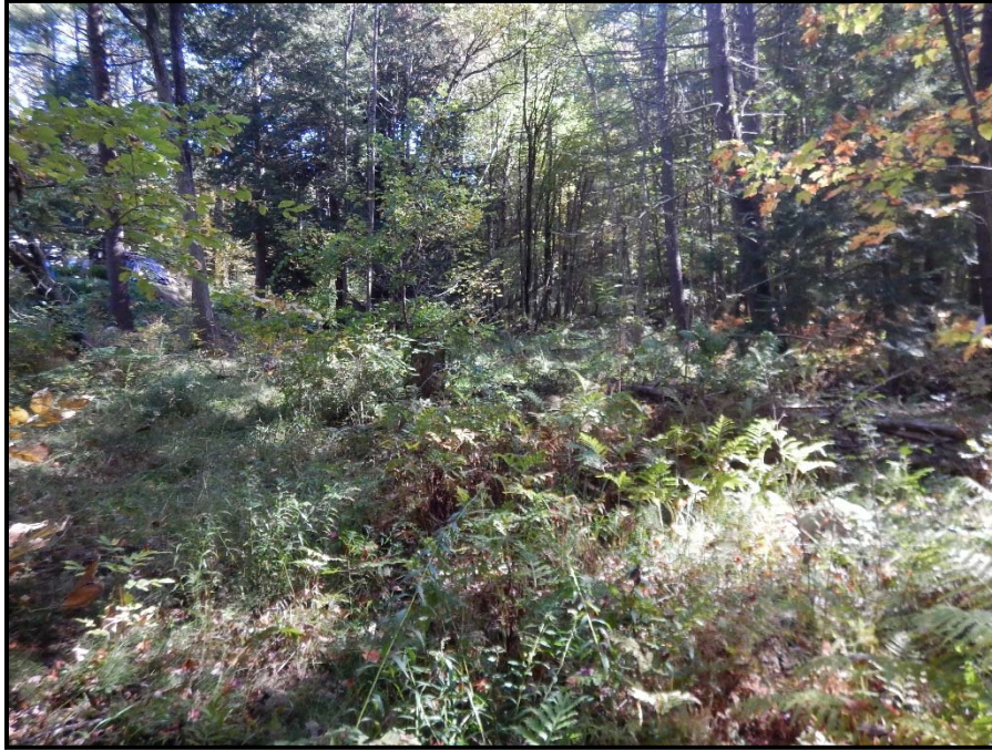
Photo 79: View south of WA 102 near location of construction work pad for pole installation outside of wetland. Tree clearing planned nearby. 10/03/2014.
