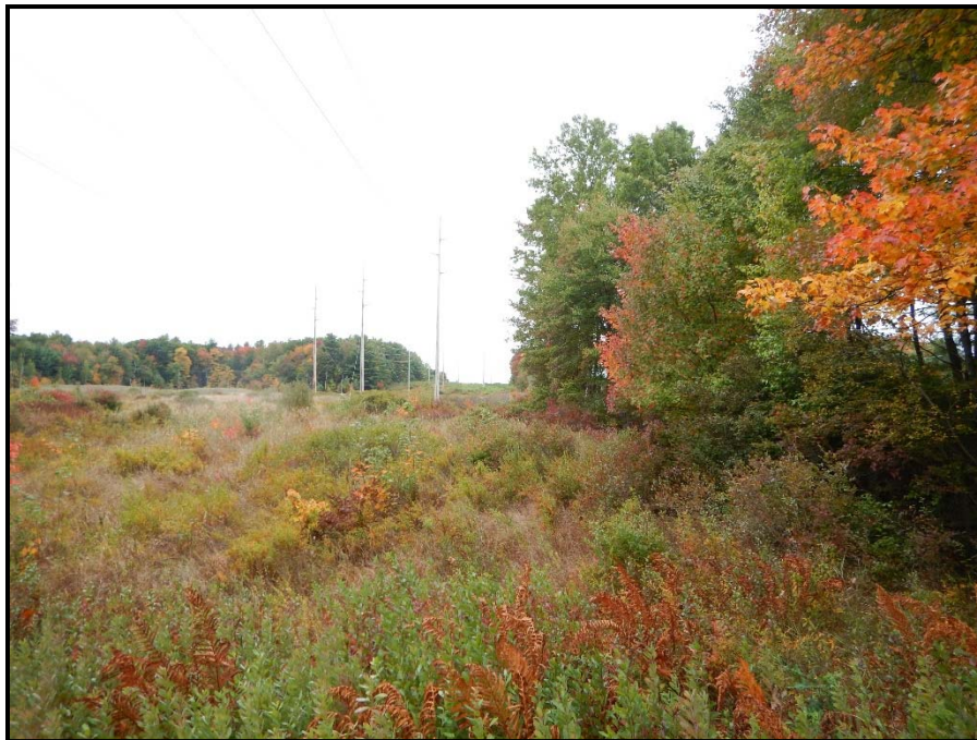
Photo 112: View west toward WA 137. To the west is the location of a construction work pad for pole installation just outside of wetland. 09/30/2014.
