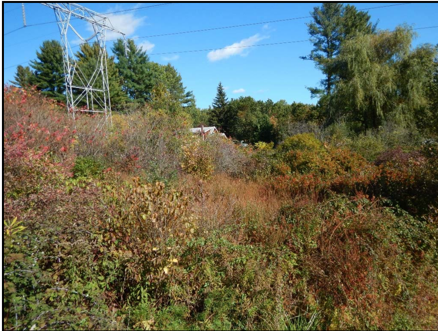
Photo 50: View north toward WA 73. Construction work pad for pole installation outside of wetland to extend into this section of the wetland. Tree clearing proposed in wetland along ROW. 10/08/2014.
