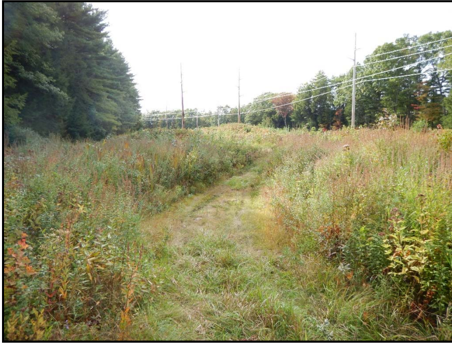
Photo 127: View west toward southern end of WA 156 along access road. Location of timber mat access. Tree clearing planned to right of photo. 09/25/2014.
