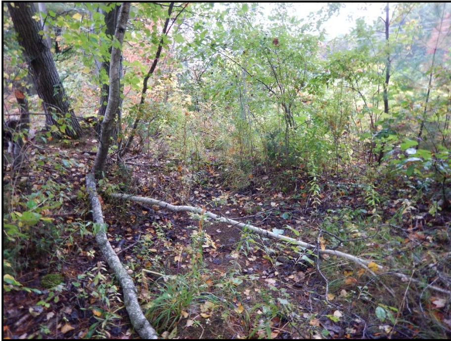
Photo 107: View southeast toward WA 128A of area where clearing is planned. General location of construction work pad for pole installation just outside of wetland. 09/30/2014.
