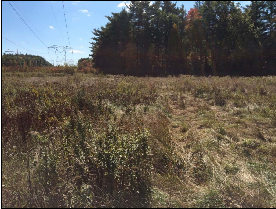
Photo 37: View southeast toward WA 54A. Two construction work pads planned near this area, one for pole installation outside wetland and one to install Structure 51 within wetland. Timber access matting planned along NEP access road into wetland. 10/09/2014.
