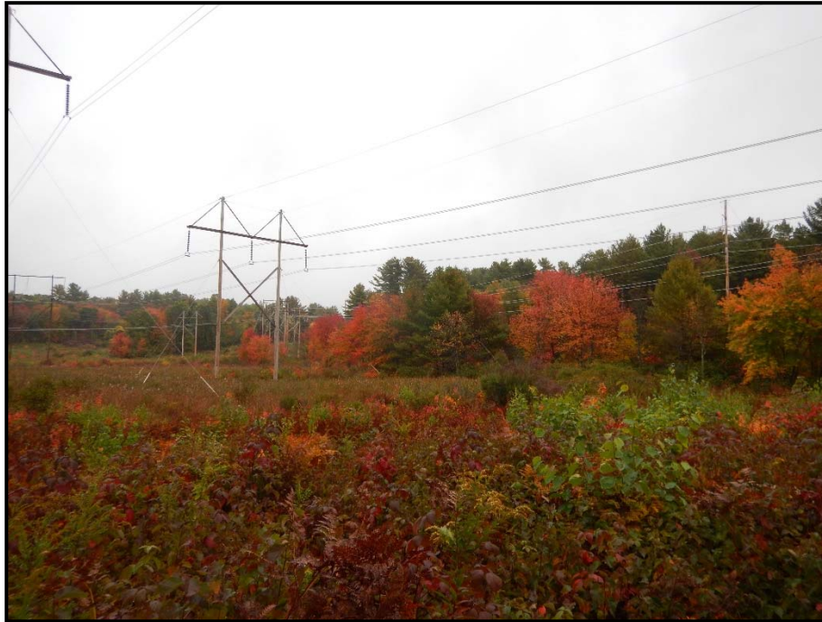
Photo 105: View east toward Eversource access road through WA 128 where timber access matting is planned. Construction work pad planned for area further east for pole installation in an upland area within wetland WA 128. Tree clearing is also planned for this area. 10/01/2014.
