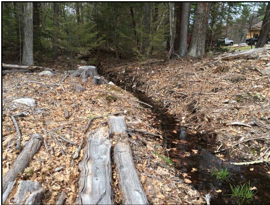
Photo 30: View west of SA-149A which flows into wetland WA 149. 04/22/2015.
