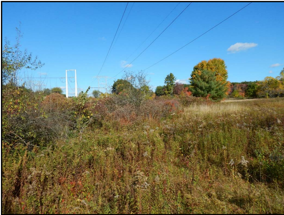
Photo 52: View north toward WA 75B. NEP access road where timber access matting is planned to right of photo. 10/08/2014.
