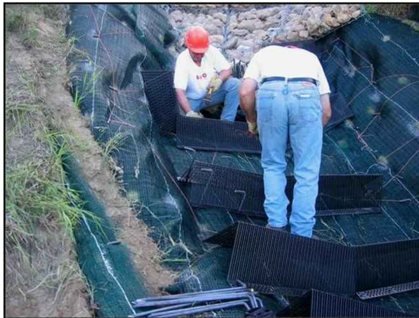
BMP # 6 EROSION CONTROL BLANKET - DITCH * (2 OF 2)
