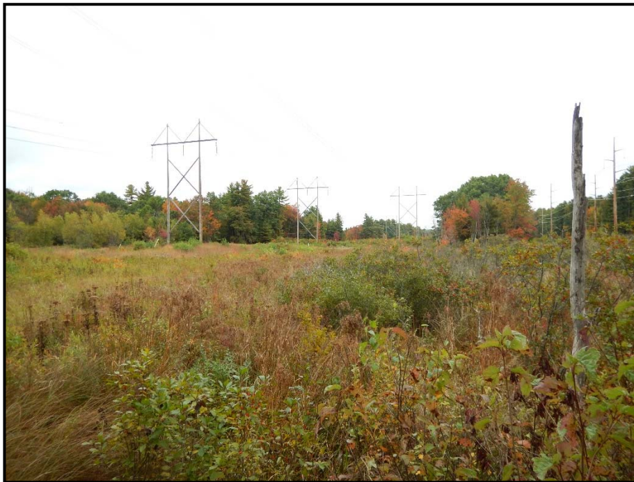
Photo 88: View northeast toward WA 110. Tree clearing planned in this area. 10/02/2014.
