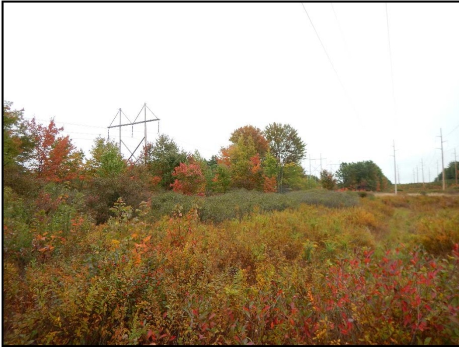
Photo 111: View east toward WA 137. Tree clearing proposed within wetland along edge of ROW. 09/30/2014.
