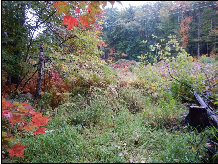
Photo 99: View northwest of WA 117B where an intermittent stream runs through the wetland. Location of construction work pad for pole installation to right of photo. Tree clearing also planned. 10/01/2014.
