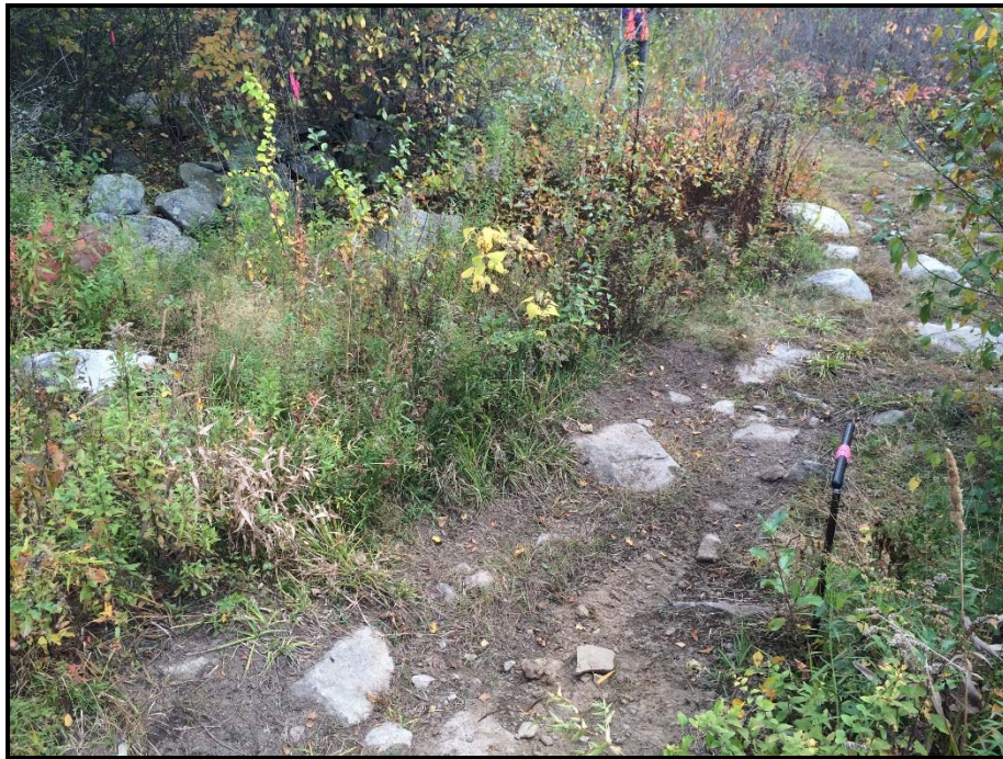
Photo 10: View southeast of access road through WA 37 where timber access matting is planned. Construction work pad for pole installation is planned just outside of wetland. 10/08/2014.
