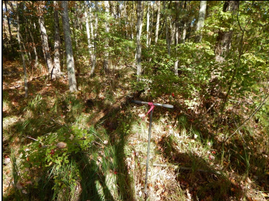
Photo 60: View west of WA 86. Tree clearing planned to the west of photo. Construction work pad for installing Structure 212 within wetland to the left of photo. 10/06/2014.
