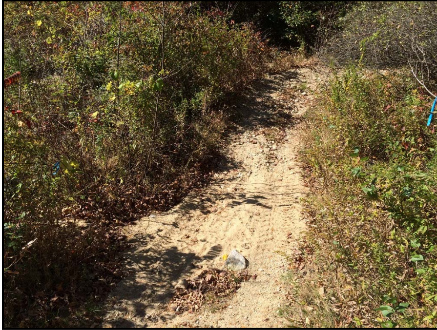
Photo 5: View northwest where timber mat access is planned along NEP access road across perennial stream SA-16. 10/09/2014.
