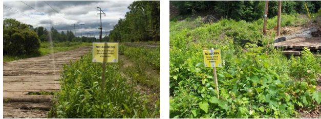
NO ACCESS – WETLAND/STREAM CROSSING MATS REQUIRED
