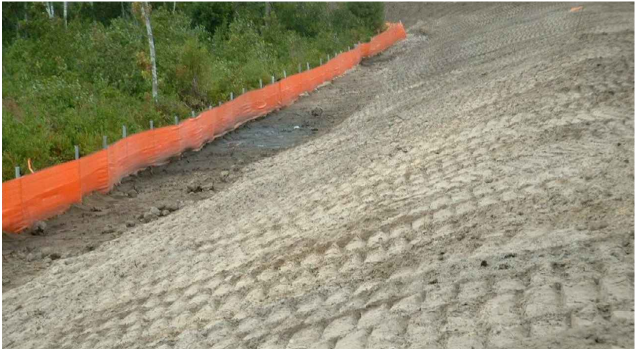
BMP # 36 BARRIER FENCE (CONSTRUCTION FENCE)
