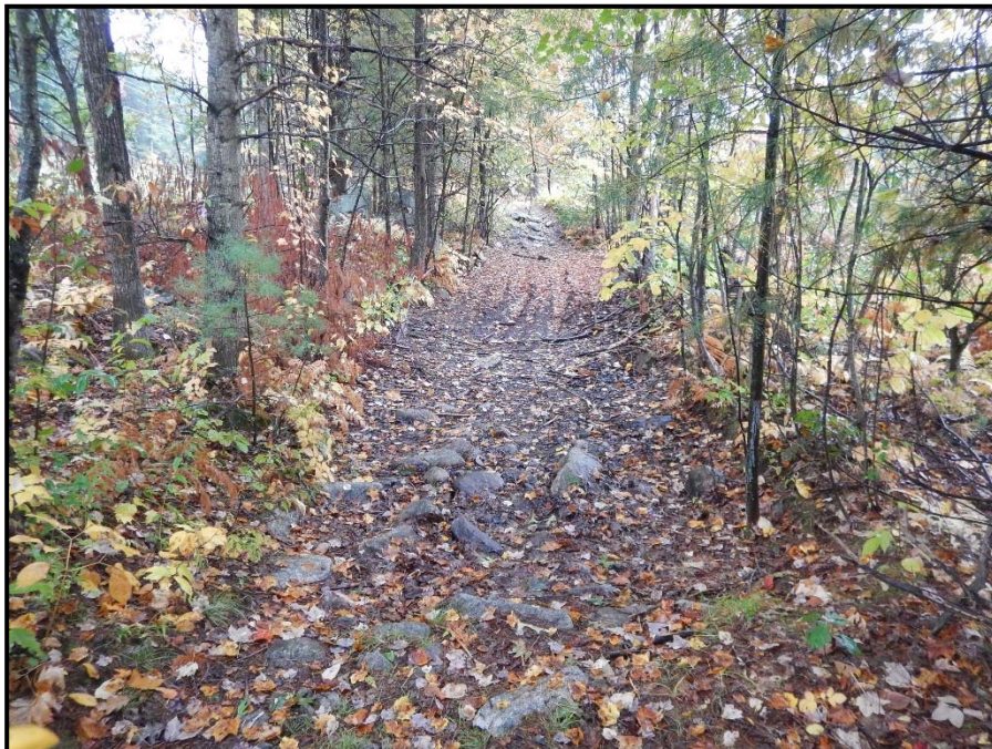
Photo 96: View southwest of Eversource access road through WA 117 where timber access matting is planned. Northeast of photo is location for construction work pad and pole installation. Pad to extend into wetland, pole to be installed just outside of wetland. 10/01/2014.
