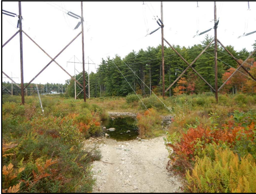
Photo 31: View northeast of ROW access road crossing perennial stream SA-43 where access matting is planned. 09/25/2014.
