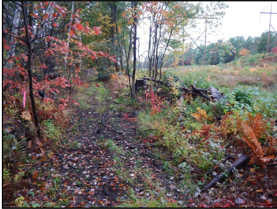
Photo 23: View south of ROW access road crossing intermittent stream SA-37 where timber access matting is planned. Tree clearing is also planned down the center of the ROW in this location. 10/01/2014.
