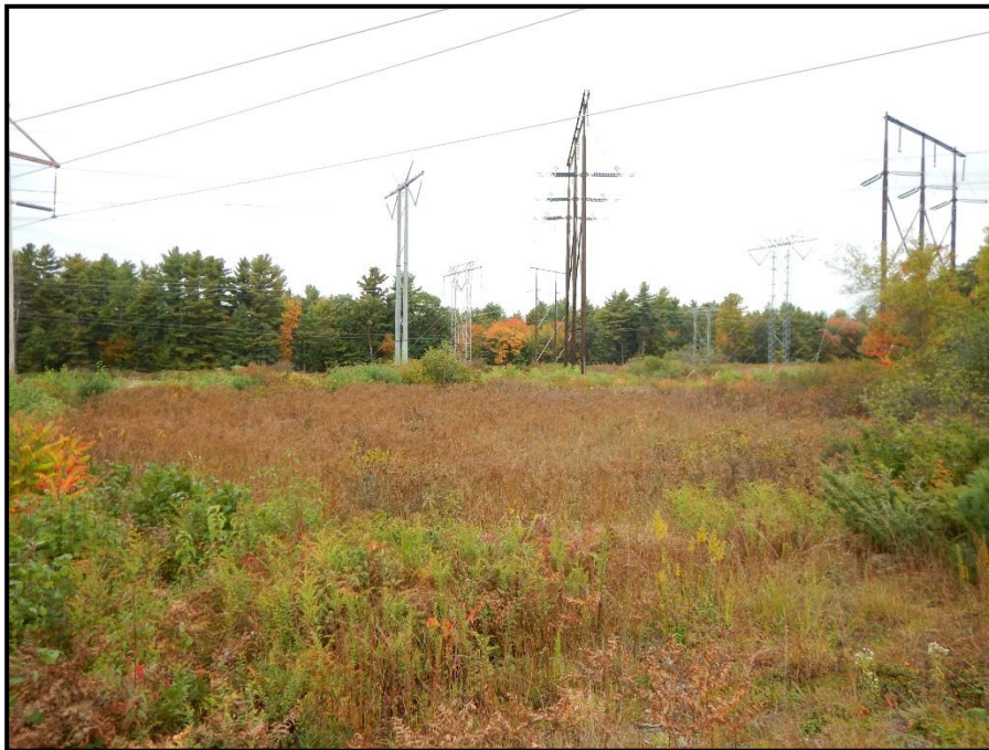
Photo 86: View west toward WA 108. Construction work pad to extend into edge of wetland as part of a large pull pad site. Guy anchor installation also proposed within this wetland. 10/02/2014.
