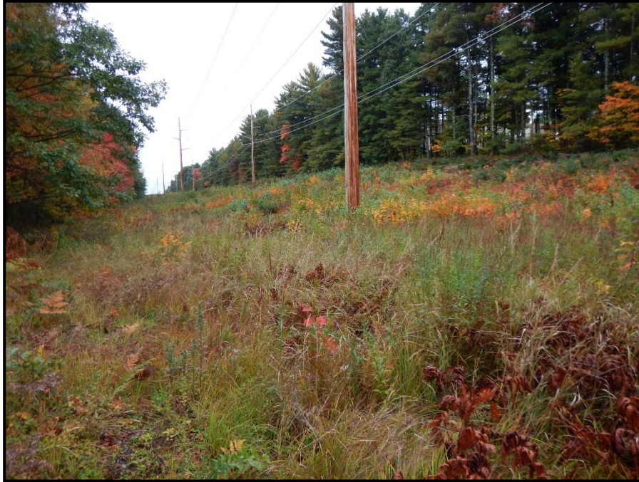
Photo 95: View northeast of WA 115. Tree clearing and construction work pad for pole installation planned to the left of photo. 10/01/2014.
