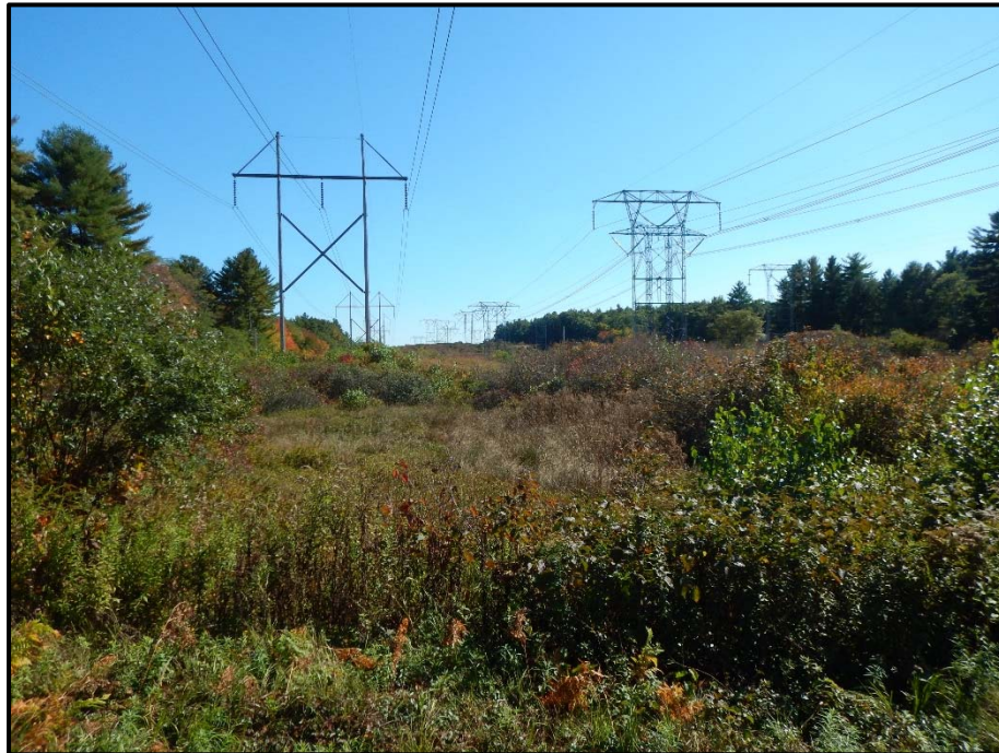
Photo 136: View southeast toward WA 87A. The eastern edge of the wetland will be temporarily impacted by a construction work pad during the installation of proposed structure 213. 10/06/2014.
