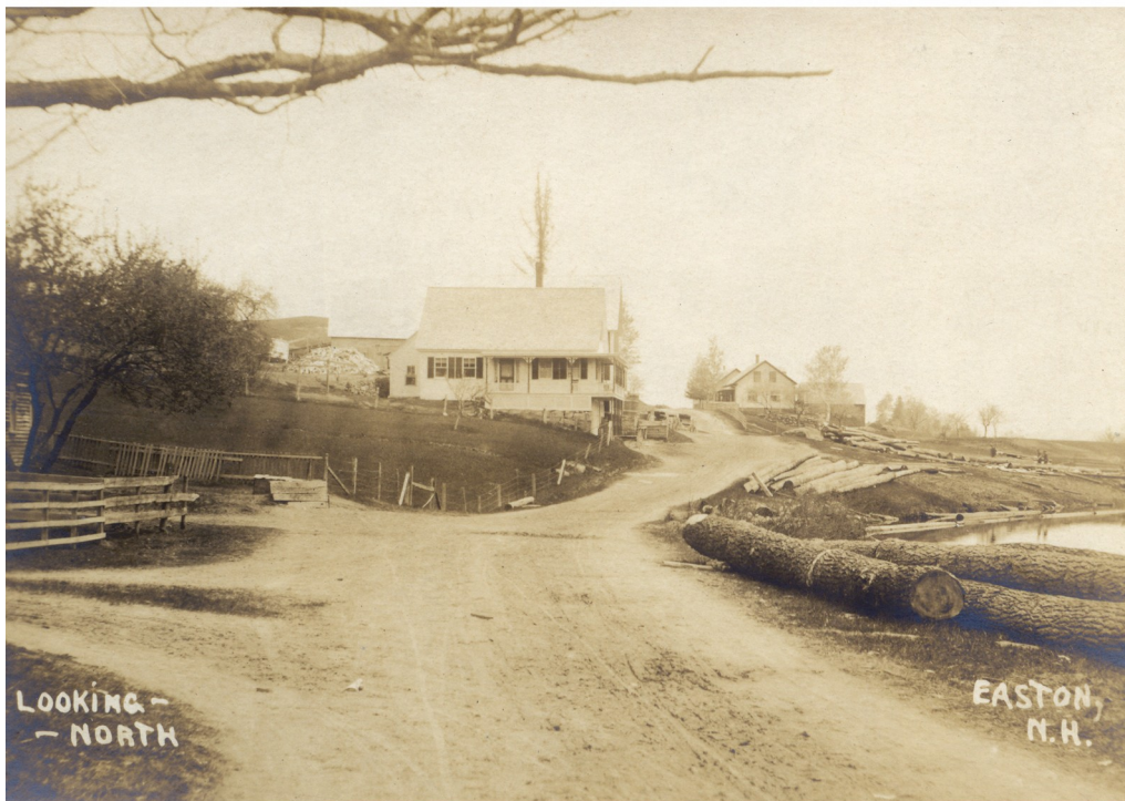
Looking North - Young's Store & Post Office on left and Daniel J. Witcher place on right.
