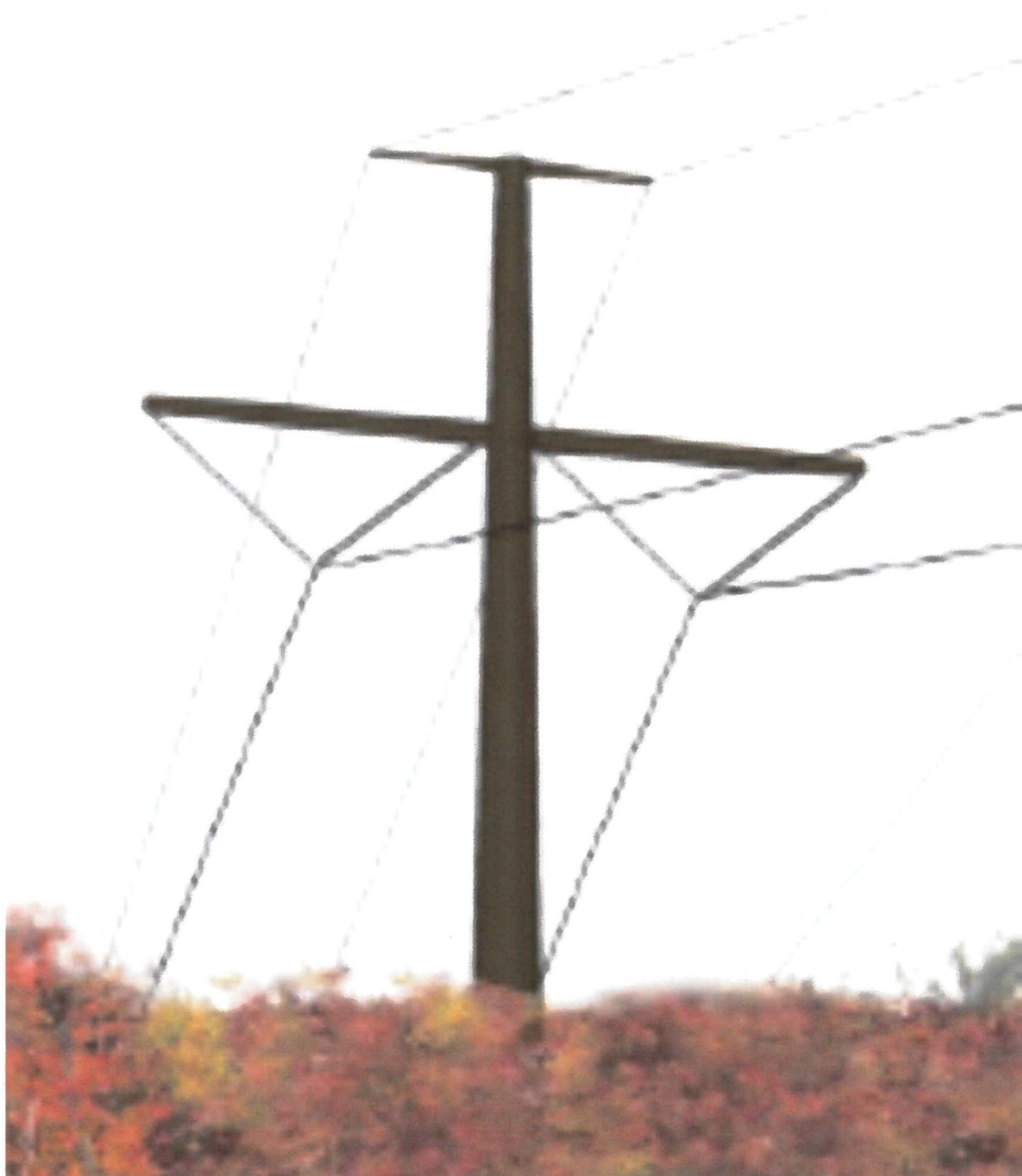
PROPOSED 65 FOOT HIGH POLE IN BRIDEGWATER ACROSS THE RIVER FROM NEW HAMPTON (From Images for New Hampton in the Northern Pass Submittal)
