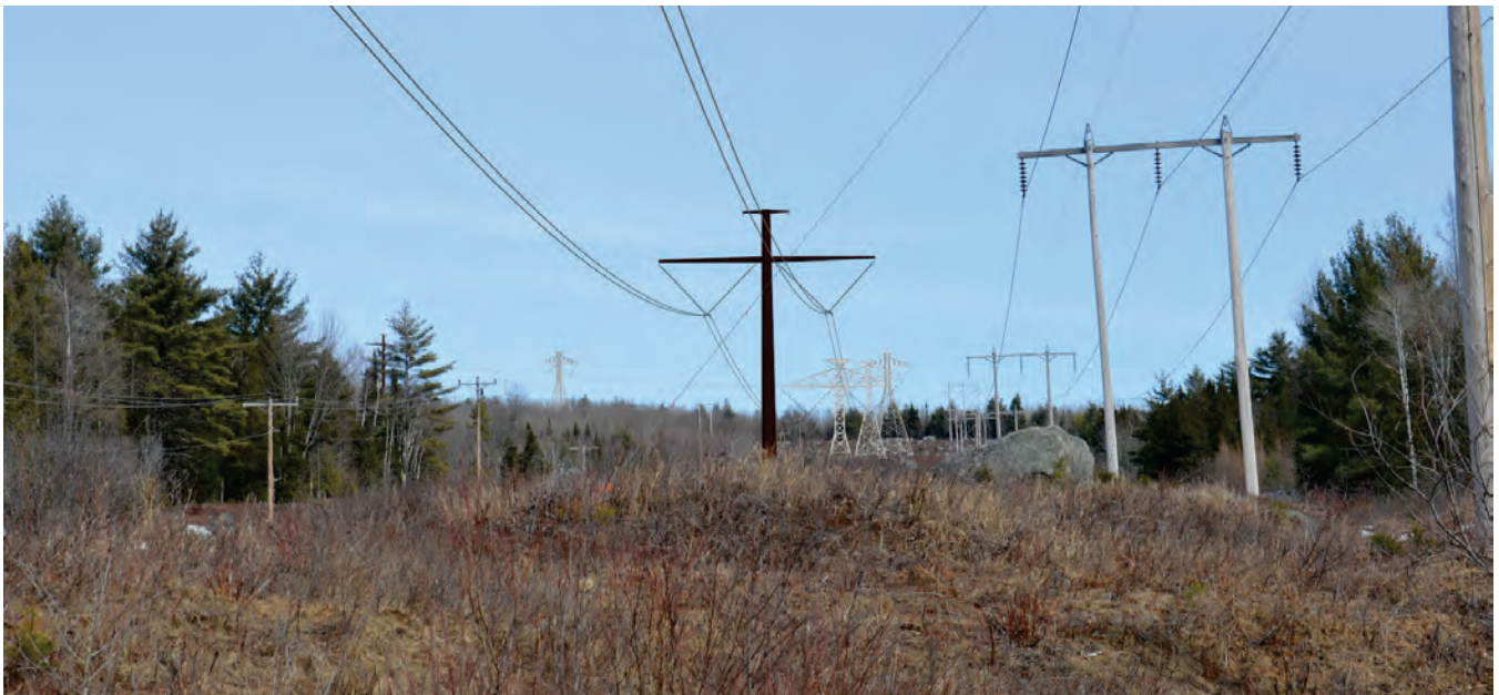
Figure 29. Cropped image simulated by T. J. Boyle where the proposed NPT crosses Route 116 in Bethlehem. Three types of transmission structures are visible in this location, including weathering steel monopoles, galvanized lattice structures, and wooden H-frame structures. Not shown is a steel monopole structure at left that would loom above the viewpoint.
