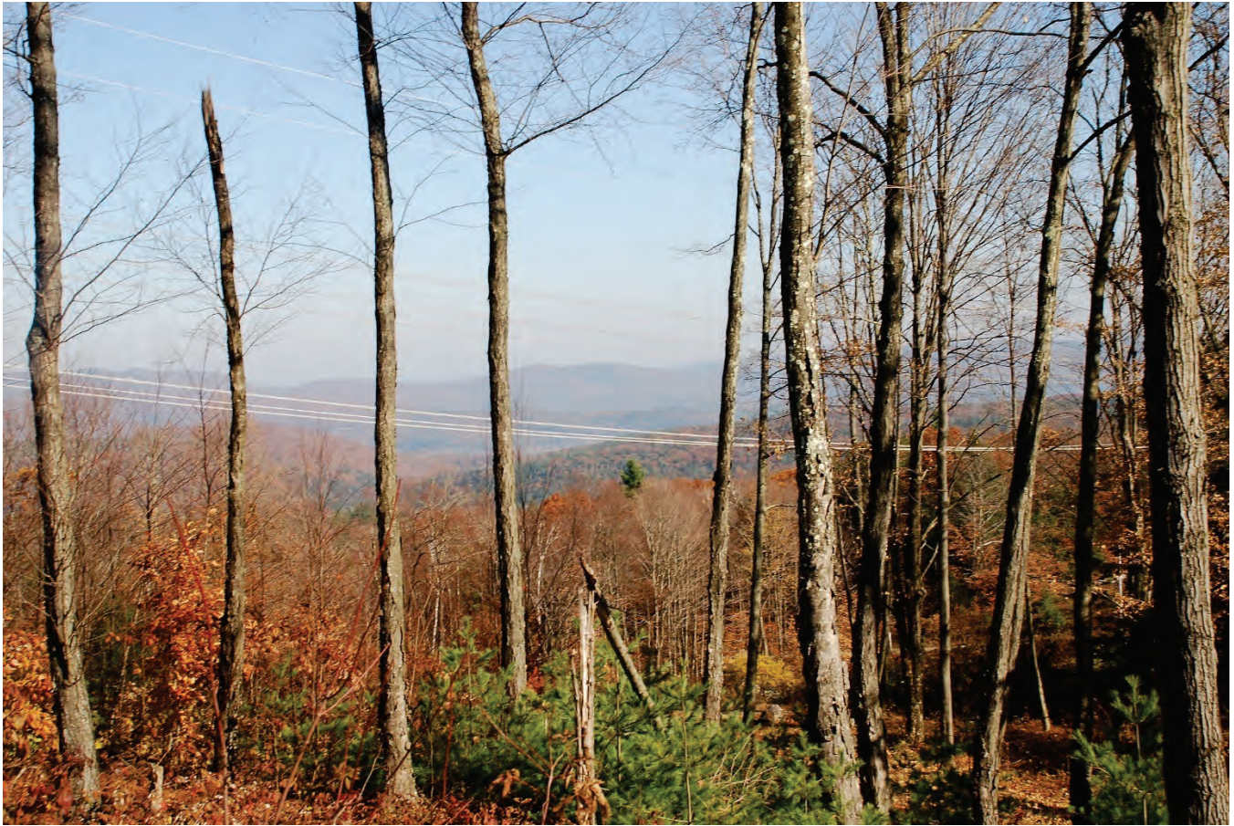
Figure 48a. Photo of the VELCO Southern Loop corridor where two 345 kV transmission lines are located in southern Vermont. The line on the bottom was installed circa 1971 using untreated conductors; the line on the top (see Figure 15b) right was installed in 2011 and used non-specular conductors. Fifty years of weathering has not eliminated the specular glare; the new transmission line with non-spectral treatment is much less visible.
