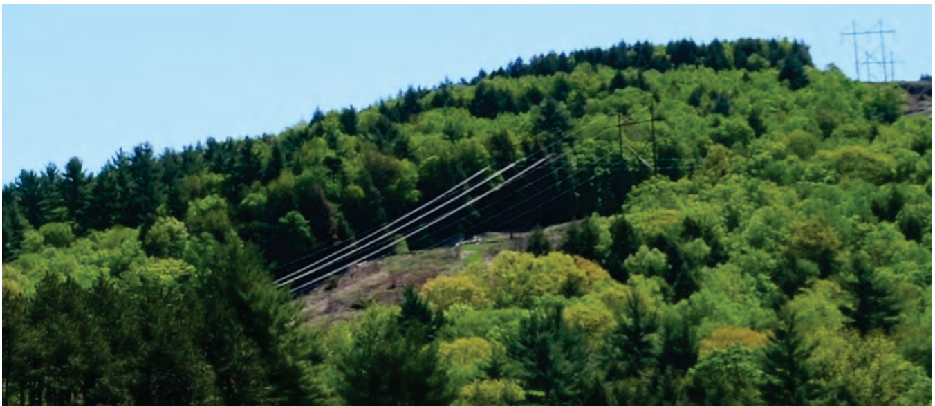
Figure 47b. Cropped photo of the photograph in Figure 14a. The line on the left was installed circa 1971 using untreated conductors; the line on the right was installed in 2011 and used non-specular conductors. Fifty years of weathering has not eliminated the specular glare; the new transmission line with non-spectral treatment is much less visible.
