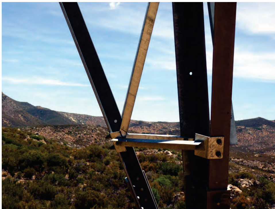
Figure 43. Close up of a galvanized steel lattice tower treated with Natina Steel.
