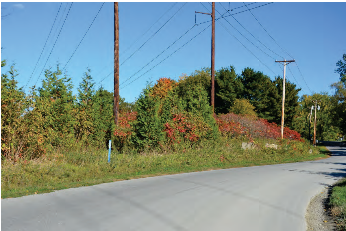
Figure 42b. Vegetation mitigation permitted and installed for the VELCO East Avenue Loop Project to screen a 115 kV corridor, after 9 years of growth. The immediate structures were not able to be screened, but the remainder of the structures in the corridor have been completely screened. Vegetation will be maintained over time to avoid clearance issues.
