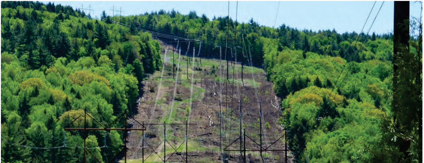
Figure 46b. Cropped photo of the photograph in Figure 13a. The line on the left was installed circa 1971 using untreated conductors; the line on the right was installed in 2011 and used non-specular conductors. Fifty years of weathering has not eliminated the specular glare; the new transmission line with non-spectral treatment is much less visible.
