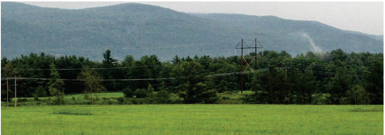
Figure 49b. Cropped portion of the photograph in Figure 16a. Even though the 345 kV transmission line uses six total conductors (top), they appear less visible than the three adjacent 115 kV conductors (bottom).
