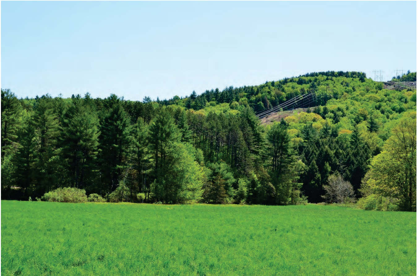
Figure 47a. Photo of the VELCO Southern Loop corridor where two 345 kV transmission lines are located in southern Vermont. The line on the left was installed circa 1971 using untreated conductors; the line on the right was installed in 2011 and used non-specular conductors. Fifty years of weathering has not eliminated the specular glare; the new transmission line with non-spectral treatment is much less visible.
