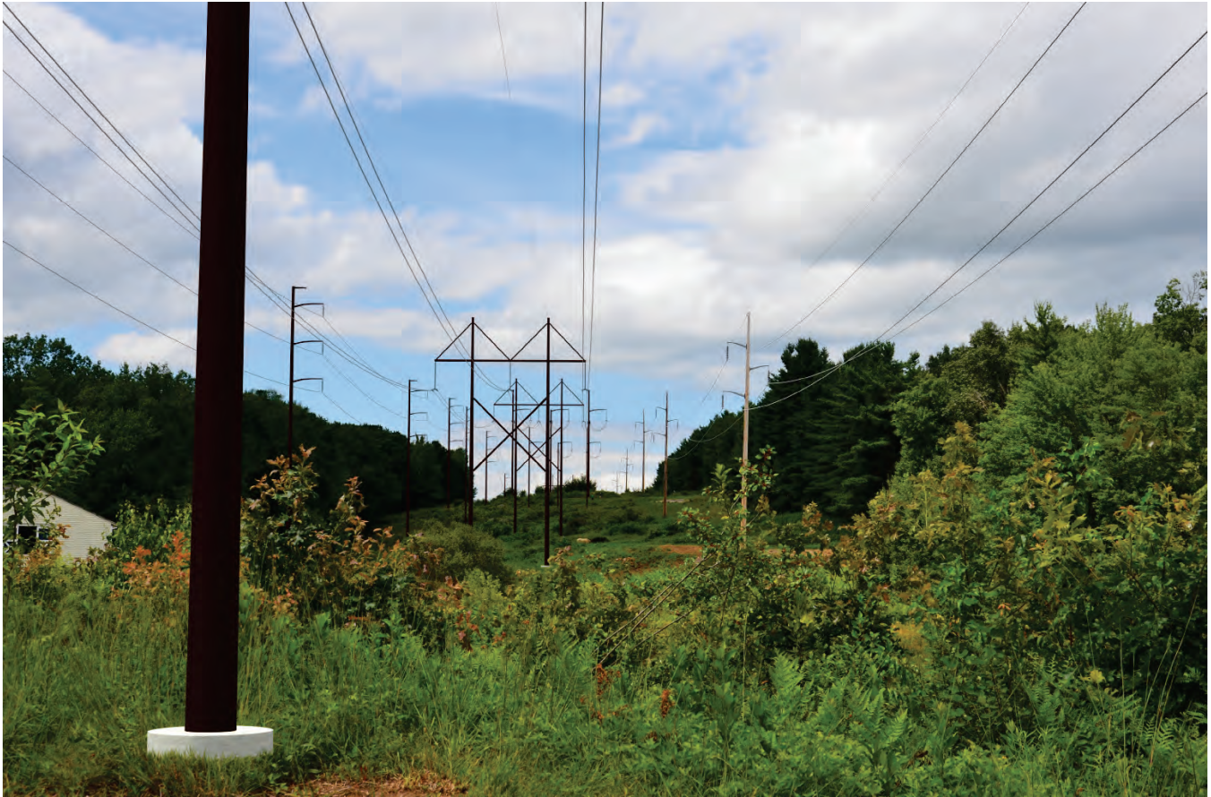
Figure 28. A simulation by T. J. Boyle where the proposed NPT crosses Route Boyce Road in Canterbury (simulation included in Appendix F at location CB-1). Three types of transmission structures are visible in this location, including 115 kV weathering steel monopoles, 345 kV weathering steel H-frames, and 115 kV wooden structures using a compact “delta” configuration. An evaluation of this location is discussed in Chapter 4.
