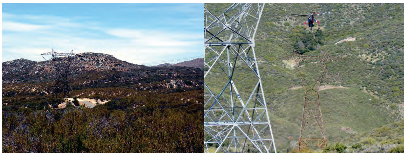
Figure 44. Left: Large galvanized steel lattice tower treated with Natina Steel. Right: Galvanized lattice structure at left compared to structures treated with Natina Steel at right. Changing the color of the galvanized lattice structures has the effect of blending the structures into the landscape.
