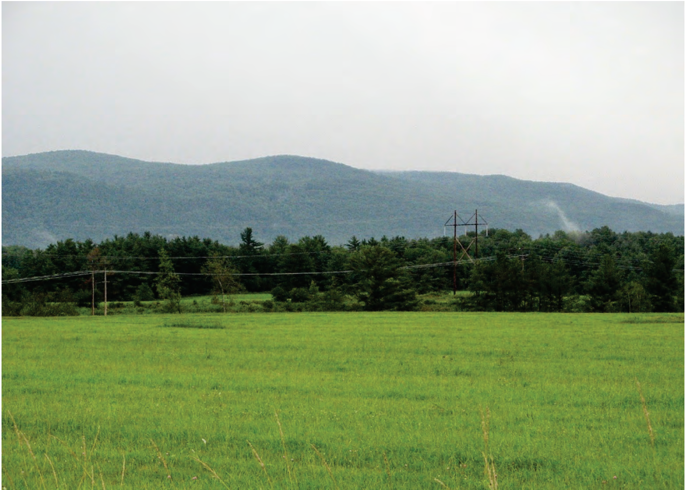
Figure 49a. Photo of the VELCO Northwest Vermont Reliability Project where a 345 kV transmission line (top) with non-specular paired conductors is located next to a 115 kV transmission line (bottom) with untreated conductors. Even though the 345 kV transmission line uses six total conductors, they appear less visible than the three adjacent 115 kV conductors.
