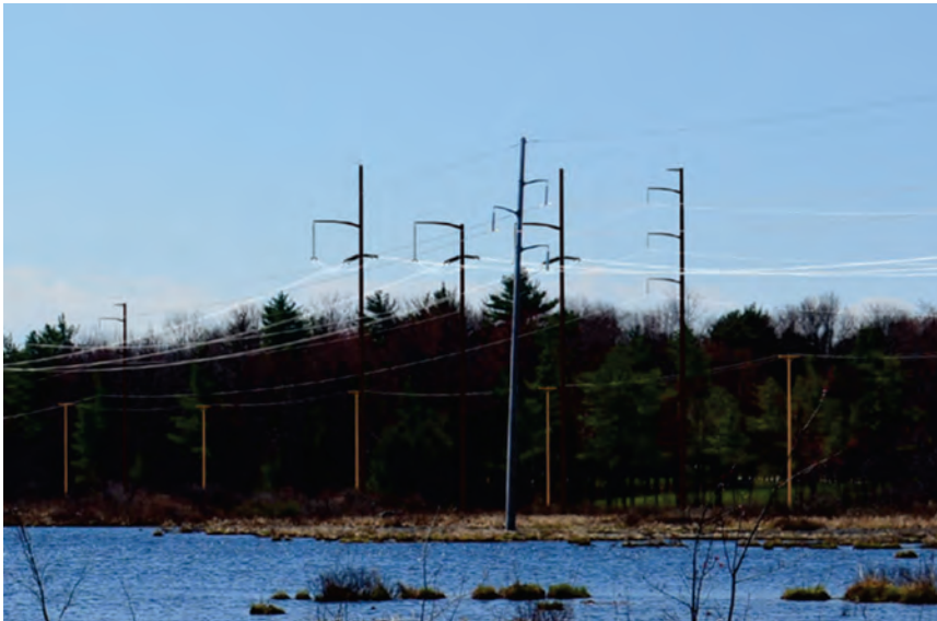
Figure 15. A cropped and enlarged image depicting the proposed three-pole structure behind the existing wooden 115-kV structure and next to the proposed weathering steel 115-kV structure. Variation in time of year, weather and sunlight affect the overall difference in color between this simulation and that shown in Figure 14. An image of Corten steel after 5-years of weathering 4 was used for the weathering steel material.
