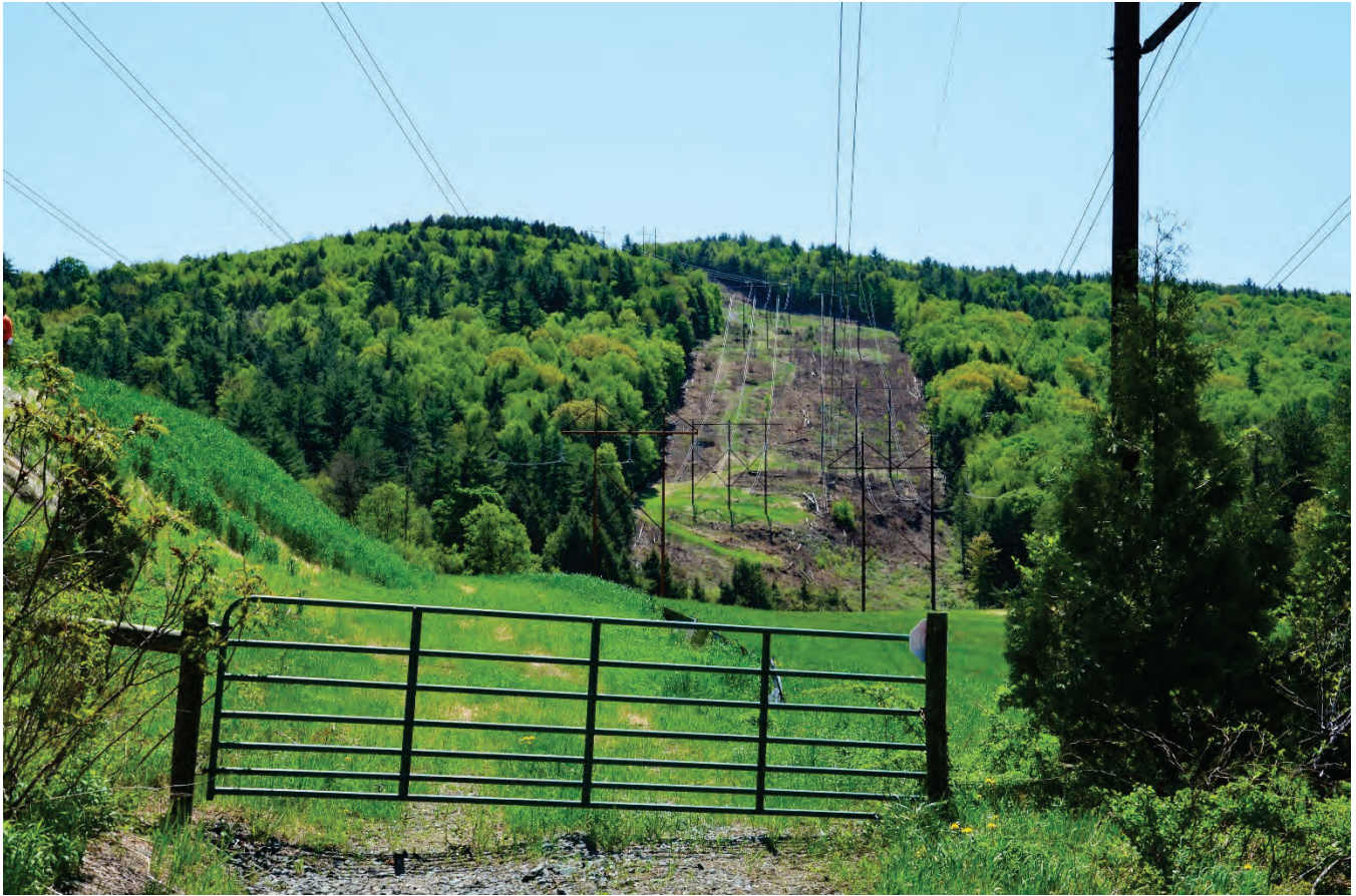
Figure 46a. Photo of the VELCO Southern Loop corridor where two 345 kV transmission lines are located in southern Vermont. The line on the left was installed circa 1971 using untreated conductors; the line on the right was installed in 2011 and used non-specular conductors. Fifty years of weathering has not eliminated the specular glare; the new transmission line with non-spectral treatment is much less visible.
