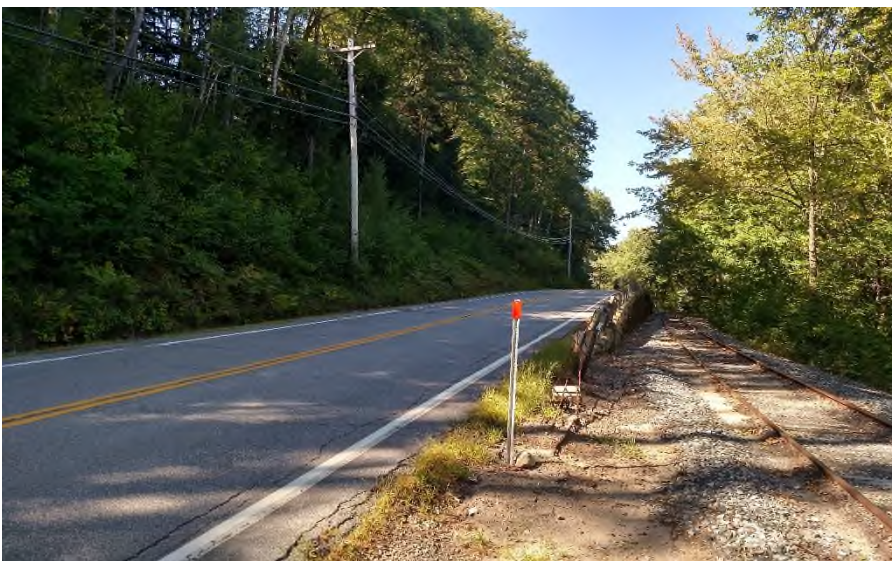
Figure 53: RT3 south of downtown Plymouth. Limited shoulder road with rock outcrops, retaining walls, steep slopes, and vegetation adjacent to road limiting construction work area.
