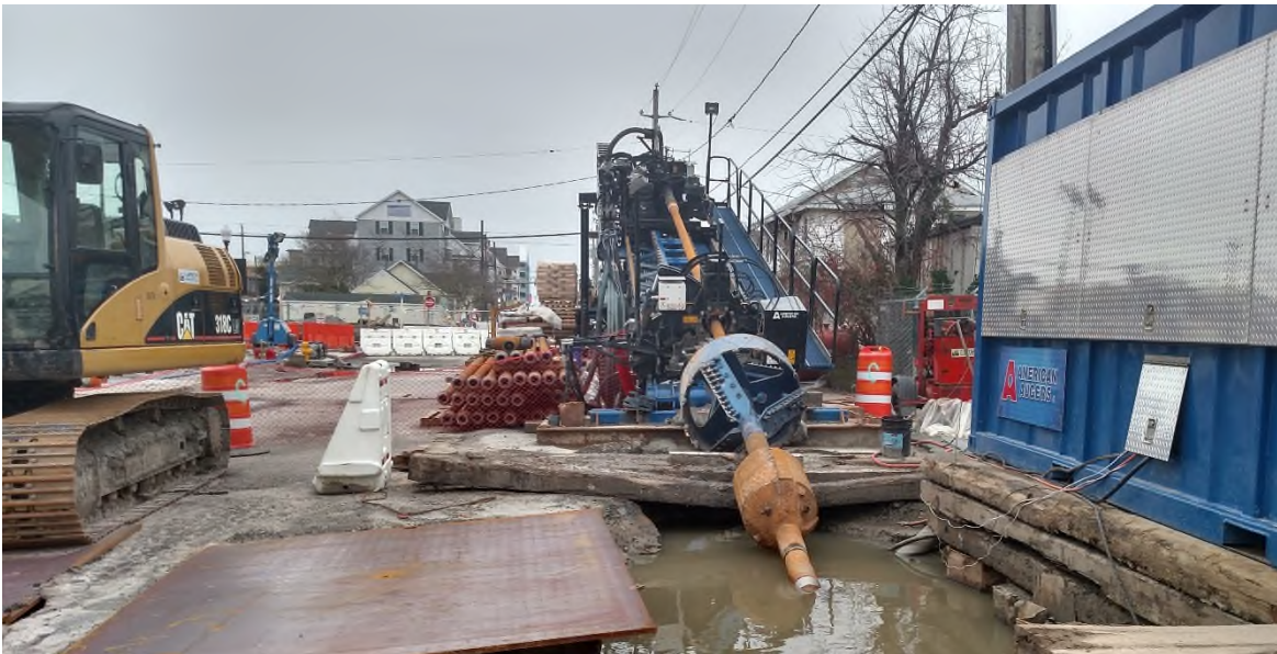
Figure 7: Example HDD drill rig and equipment set up in public right-of-way.
