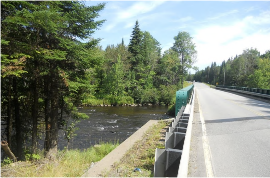
Figure 30: RT3 Bridge at Connecticut River looking north- trenchless HDD RT03 crossing proposed. HDD entry pit will be south of the bridge on the right side of Route 3 and the exit pit will be north of the bridge on the left side of Route 3 in the photo background.
