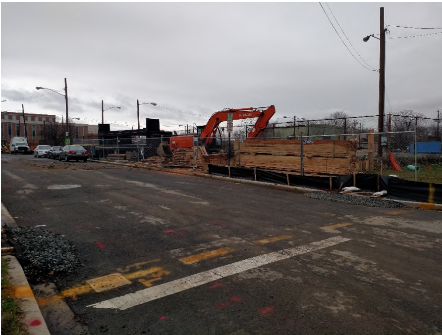
Figure 15: Excavator digging pit to prepare for trench box placement for concrete vault installation.
