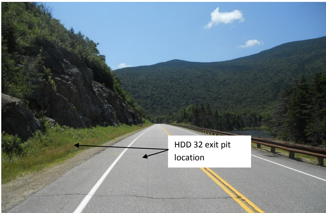
Figure 39: RT112/Lost River Road, White Mountain National Forest HDD 32- road with limited shoulders, confined by rock outcrops and guardrail. Construction will be in close proximity to Beaver Pond, shown in the right side background.
