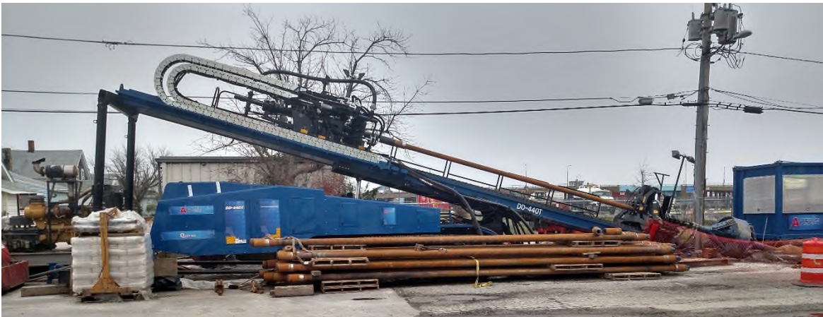
Figure 6: Example HDD drill rig and equipment set up in public right-of-way.
