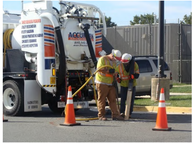
Figure 3: Utility designating Level A- vacuum excavation (photo by Accumark).
