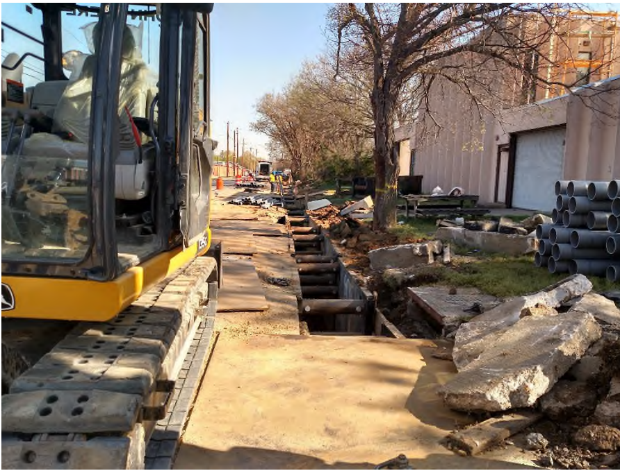
Figure 22: Example of open trench construction in urban setting with trench boxes and steel plates set aside for daily work.
