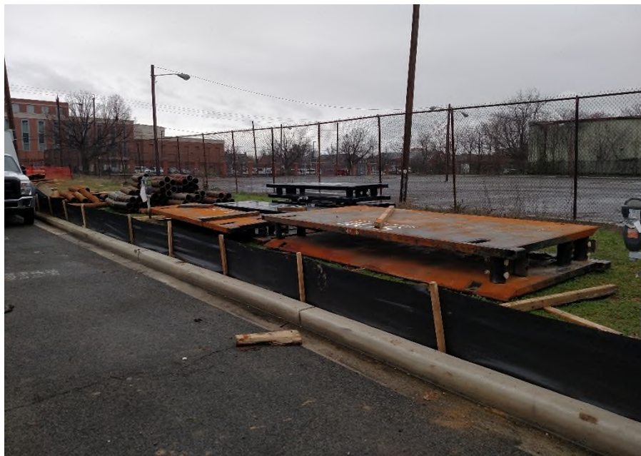
Figure 14: Trench box materials and perimeter sediment and erosion control measures.
