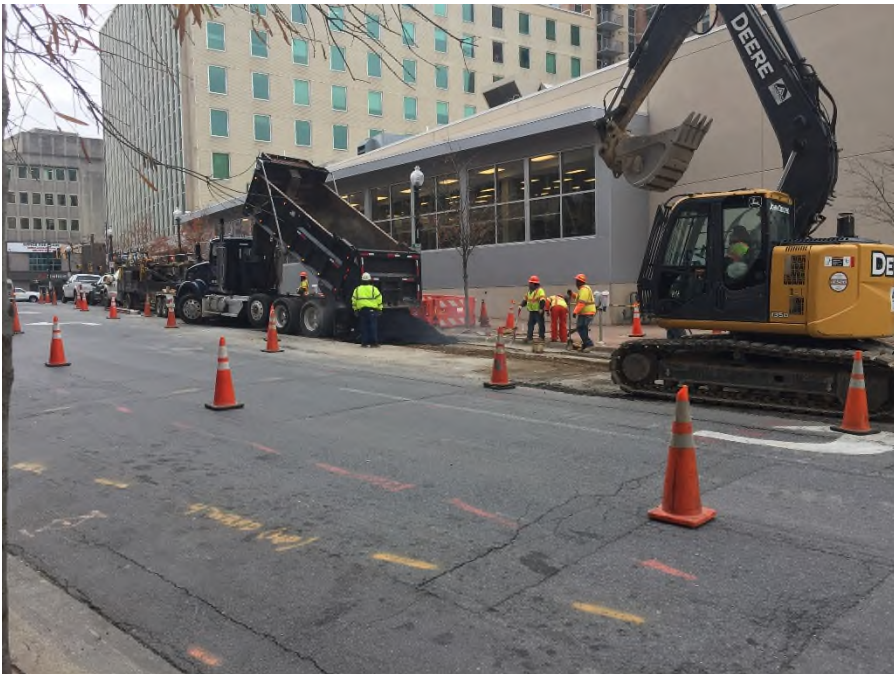
Figure 27: Example of temporary asphalt being placed at open trench construction.
