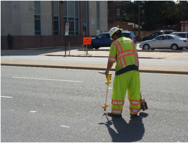
Figure 2: Utility designating Level B (photo by Accumark)
