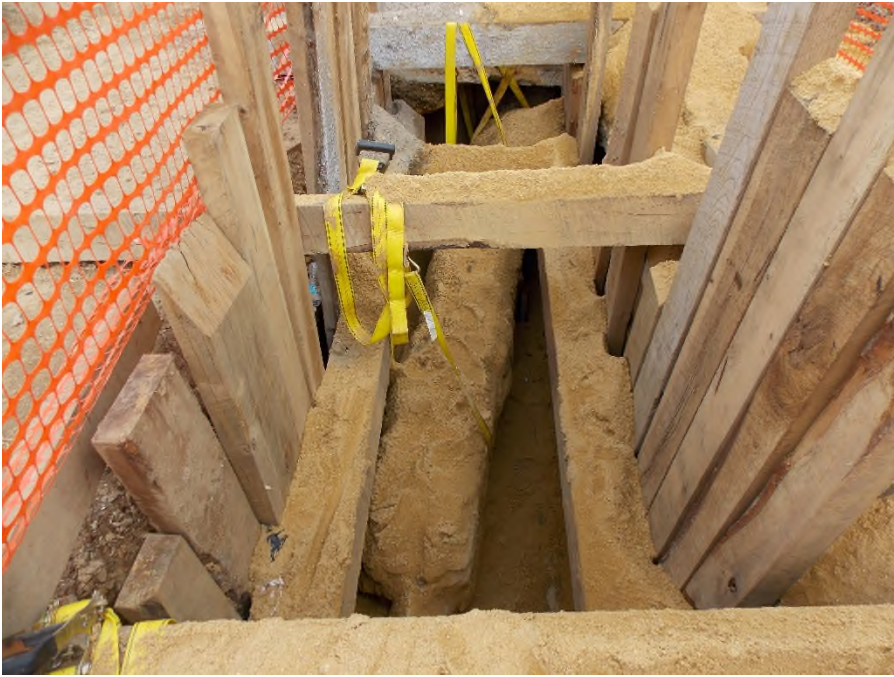
Figure 26: Example of shoring and bracing for existing underground utility above proposed underground transmission line alignment.
