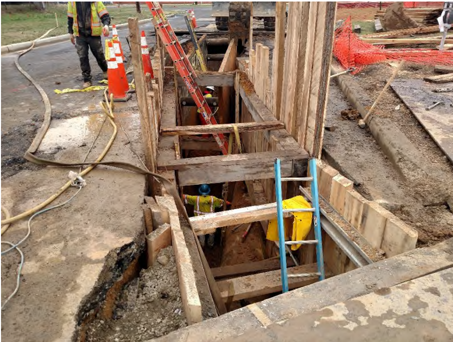
Figure 25: Example of open trench construction with shoring and bracing around existing storm drain to allow underground transmission line to traverse under the existing utility. Excavator is shown in the background.
