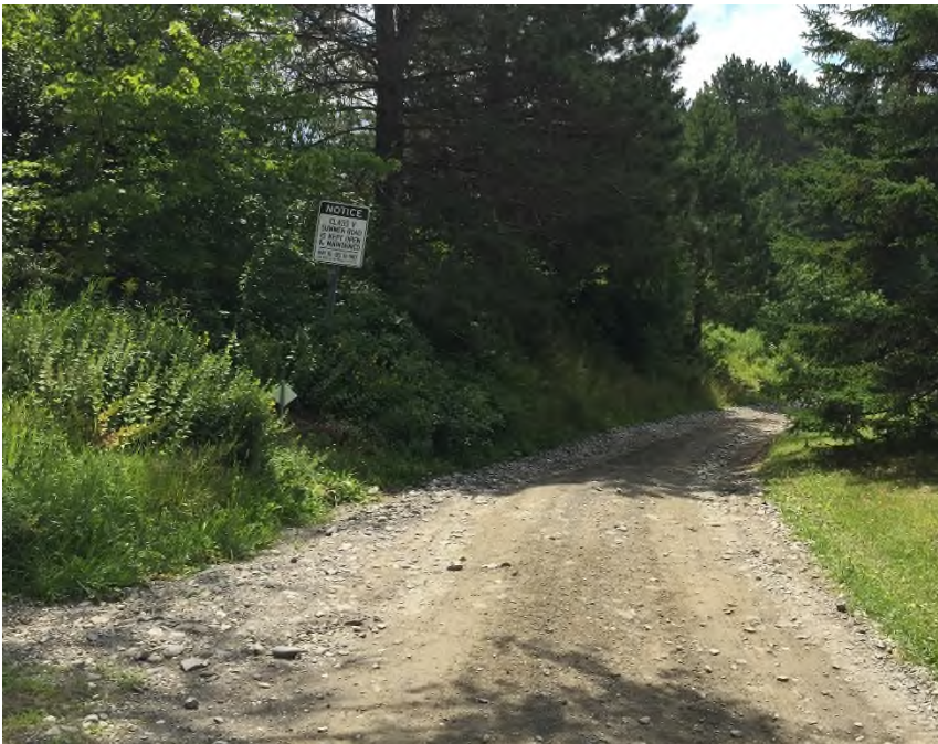
Figure 12: North Hill Road-narrow roadbed with vegetation and steep slopes adjacent to road. Trenches and splice vaults to be installed within the roadbed.
