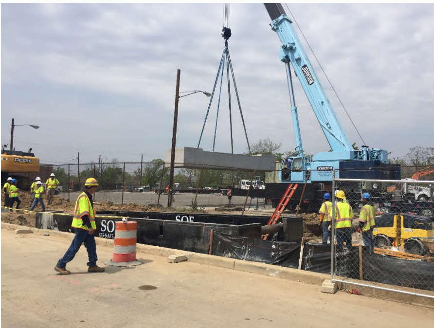
Figure 16: Crane hoisting concrete vault (~30'L x 8'W x 8'D). Compactor (yellow and black) is to the right in the photo. Excavator is to the left in the photo.
