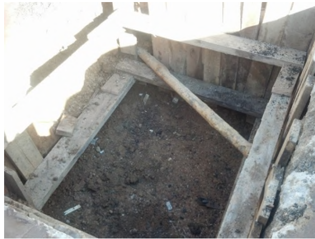
Figure 4: Utility designating Level A- hand dug test pit.
