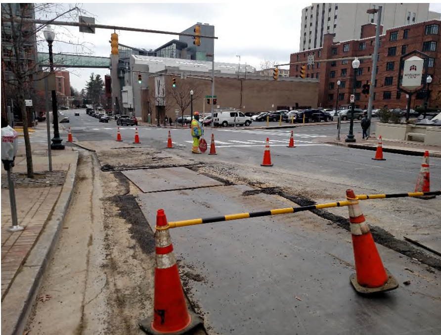
Figure 5B: Example of steel plates over open trench, traffic control cones and flagger for directing traffic.
