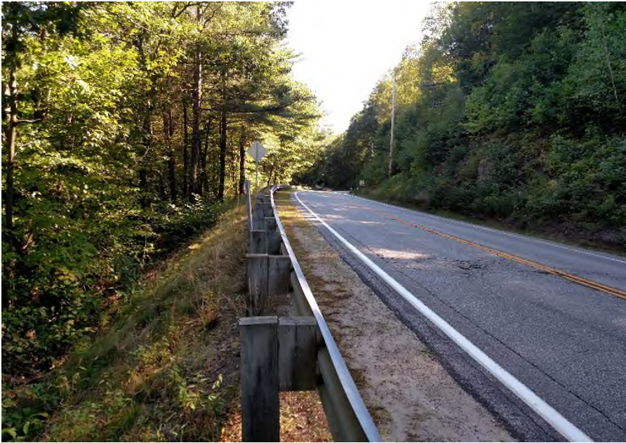
Figure 52: RT3 just south of downtown Plymouth at Parker Street. Limited shoulder road with rock outcrops, steep slopes and vegetation adjacent to road limiting construction work area.
