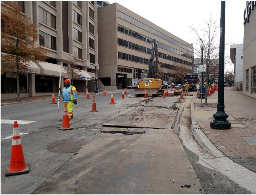
Figure 24: Example of steel plates covering open trench work at the end of work day.
