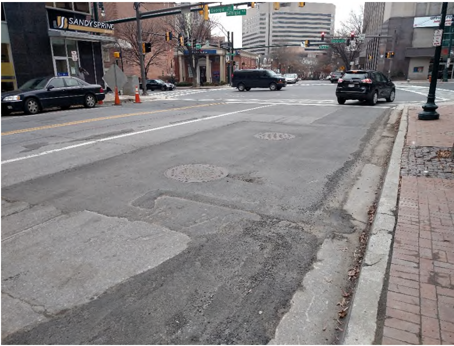
Figure 28: Example of temporary asphalt patch at vault and duct bank trench within roadbed.
