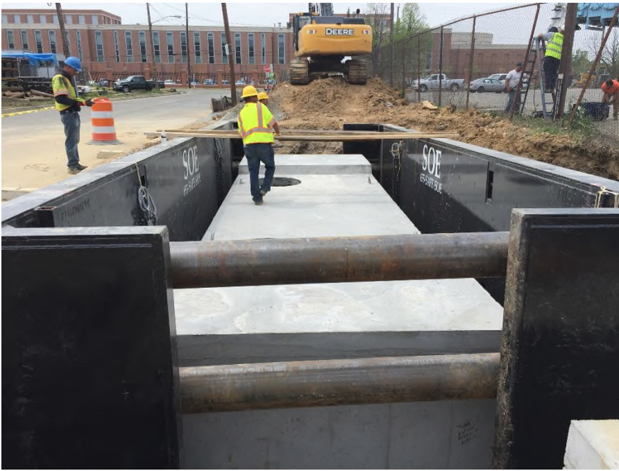
Figure 17: Precast concrete vault after placement inside trench box. Excavator is in the background.
