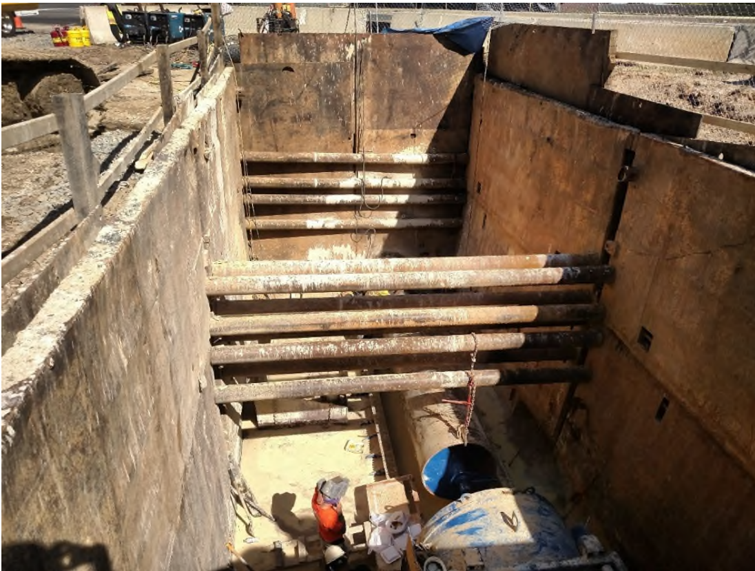
Figure 9: Example Jack and Bore set up with 20'W x 40'L x 20'+D pit. Pit maintained with trench boxes. Steel casing in middle ground and jacking rig in lower foreground.
