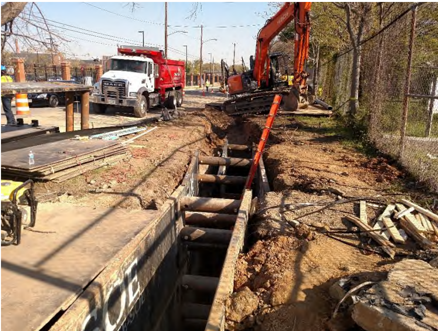
Figure 23: Example of open trench construction with one lane traffic closure adjacent to trench outside of road area. Excavator, dump truck, trench box, steel plates, generator and traffic barrel shown.
