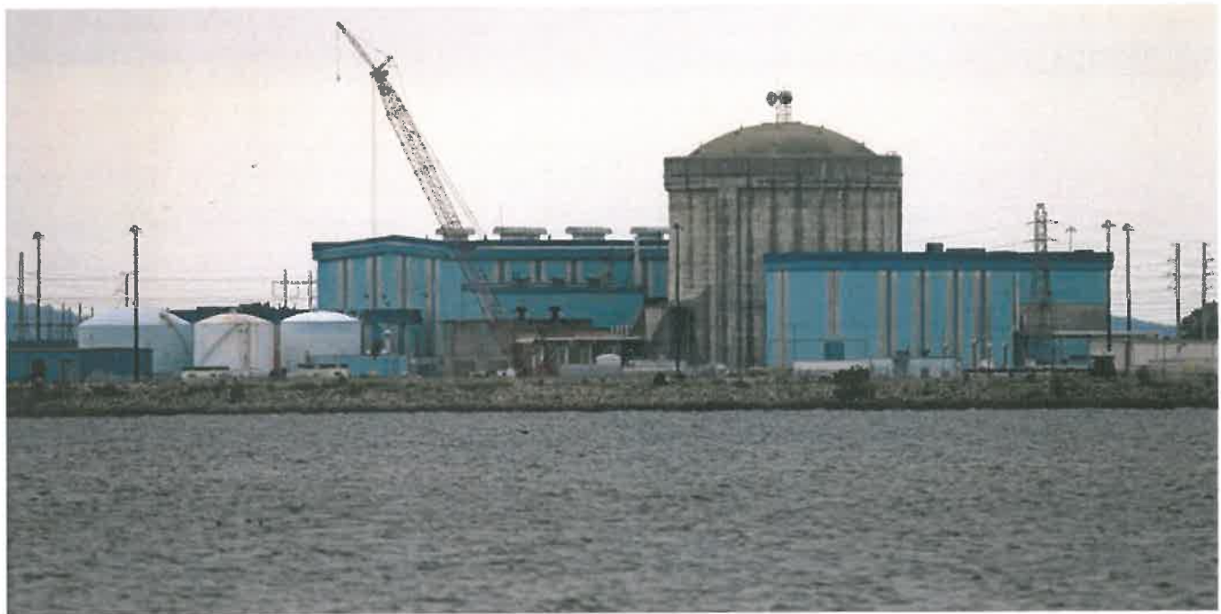
Unit one of the V.C. Summer Nuclear Stations near Jenkinsville, South Carolina, in 2106. Chuck Burton / AP
