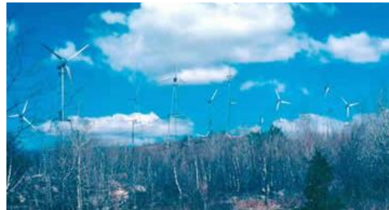
Above photo: Wind farm on Crotched Mountain in Greenfield, NH. In December of 1980, US Windpower installed the world's first wind farm, consisting of 20 wind turbines rated at 30 kW each. For a variety of reasons, including unreliable equipment and poorly understood wind resources, the project was not a commercial success and dismantled after a year.
